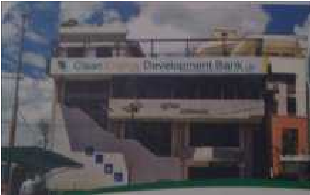
Figure1: Clean Energy Development Bank, Head office Sitapaila.
