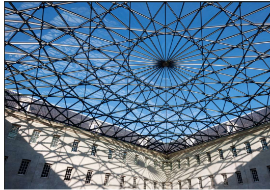
Figure 2 Grid Shell - Glass roof Dutch Maritime Museum ( Glass roof Dutch Maritime Museum at Amsterdam, Netherlands , 2017)
