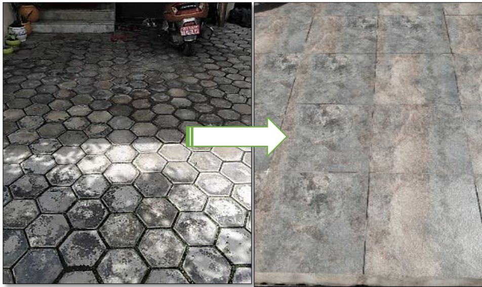
Figure 4.28 Parking tiles changed from cement blocks to Vitrified Tiles
