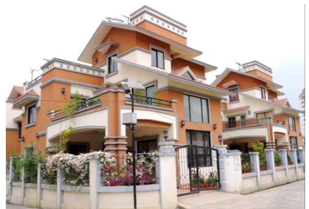
Figure 3.3 Civil homes phase 6
