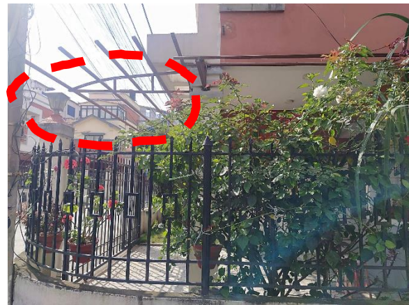
Figure 4.51 Addition of sun shading at the porch being newly constructed
