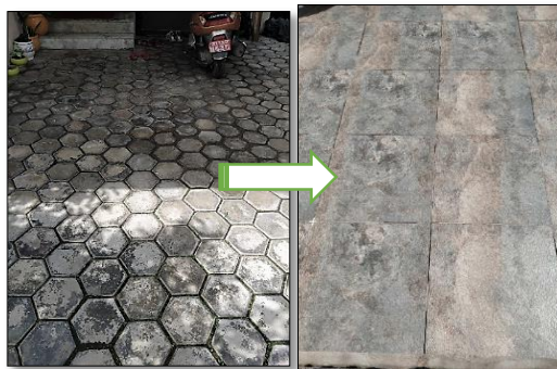
Figure: concrete block parking tiles changes into vitrified parking tiles
