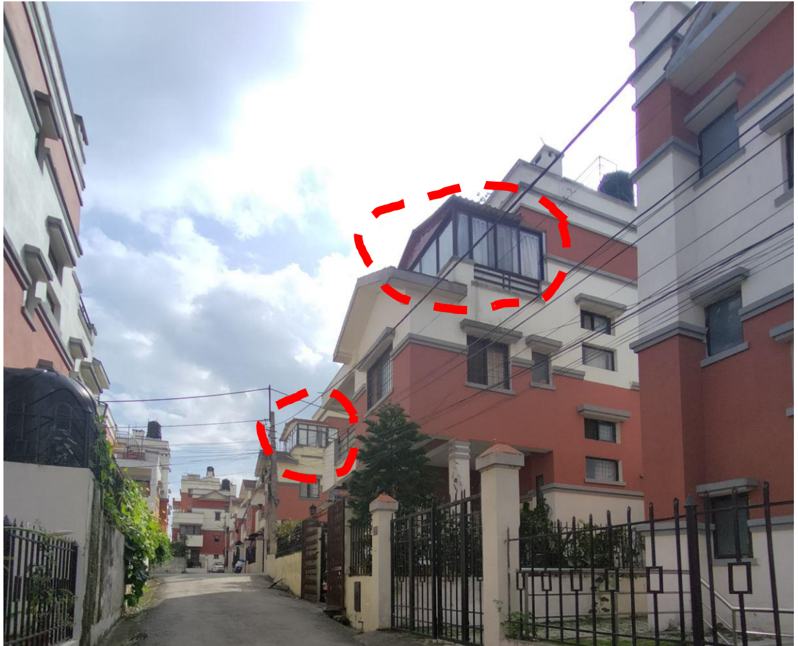
Figure 4.54 Addition of temporary structure at terrace
