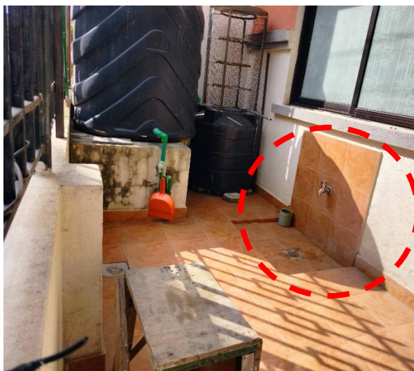
Figure 4.61 later added tap outside the building
