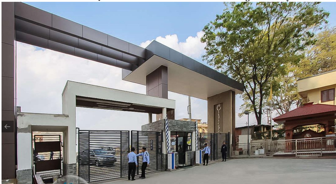
Figure 4.35 Heavy security at the main gate of housing community
