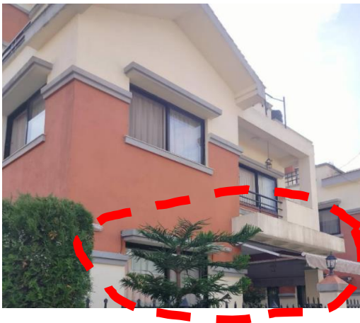
Figure 4.50 Temporary shading at the front of house
