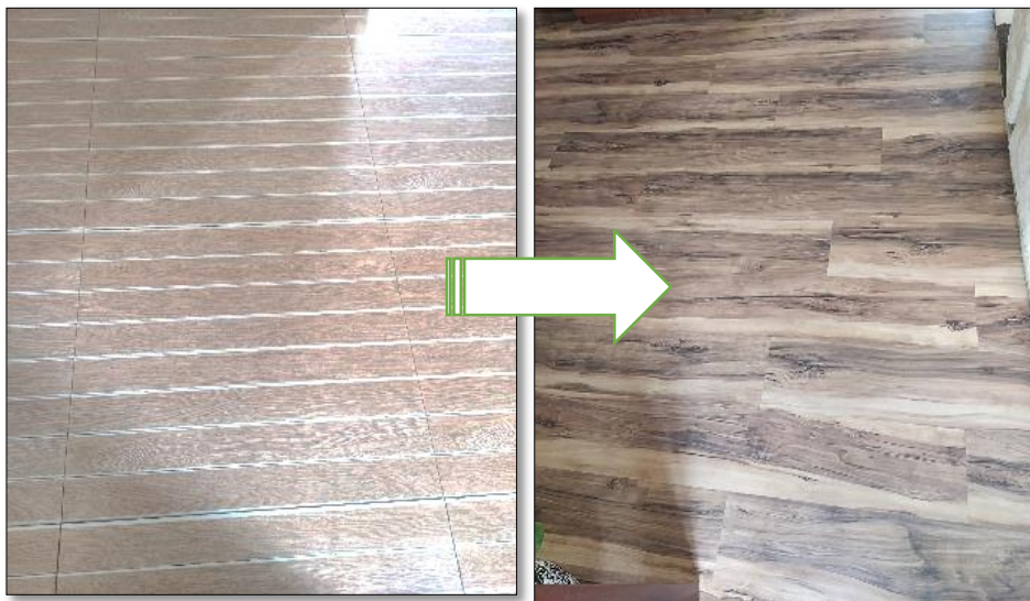
Figure 4.27 Interior floor finish material changed to parquetting from ceramic tiles
