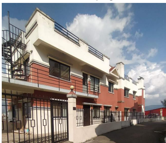
Figure 4.55 Sunlight entering inside building till late afternoon
