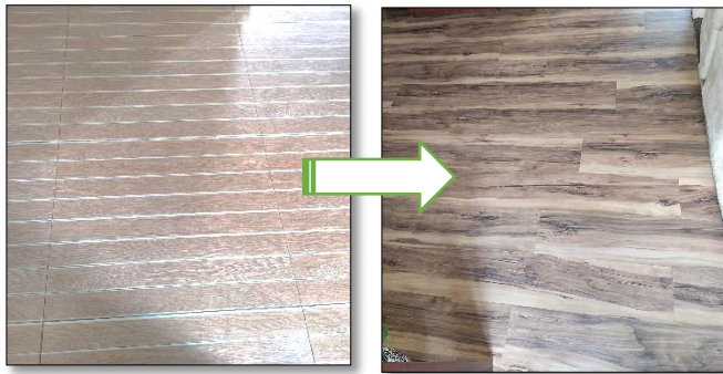
Figure: flooring material changed from tiles to parquet
