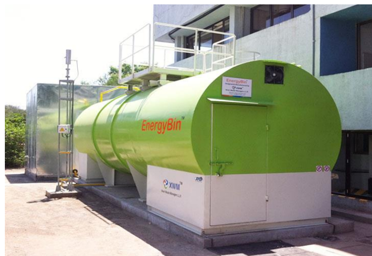
Figure 2.1: Model: EB-1000 Waste Capacity: 1,000kgs/Day Weight of the Plant: 18 Tons
