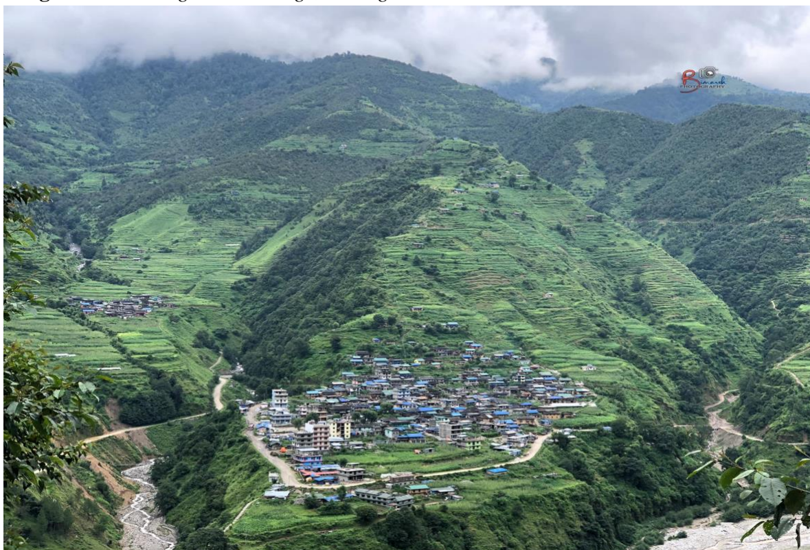
Figure 2: Thabang, Main Village, Thulagaun
