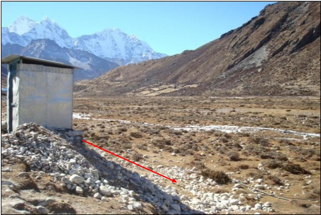
a) Toilet on the bank of Lobuche river of Pheriche.
