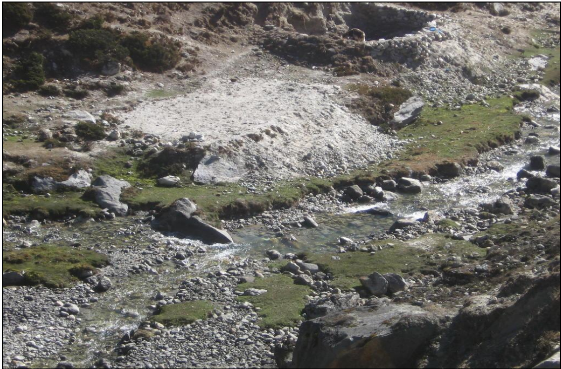
a) Constructing of garbage pit near the water course.
