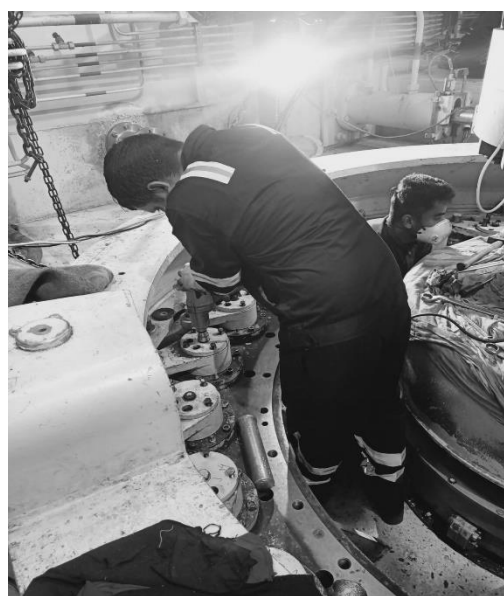
Repair of Guide Vanes
