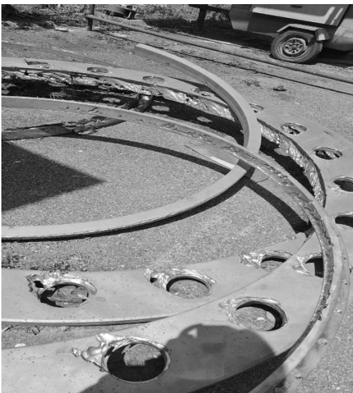
Damaged Facing Plates
