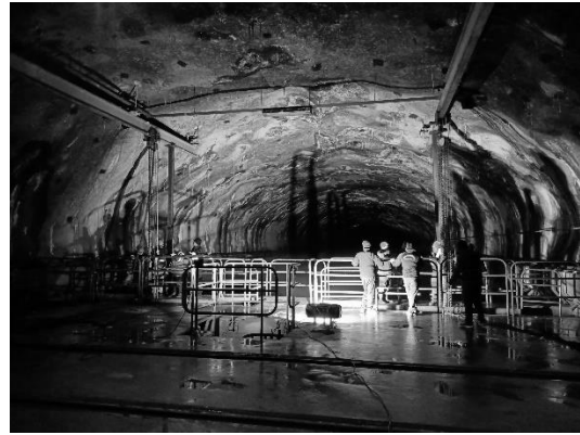
Desander Basin Maintenance
