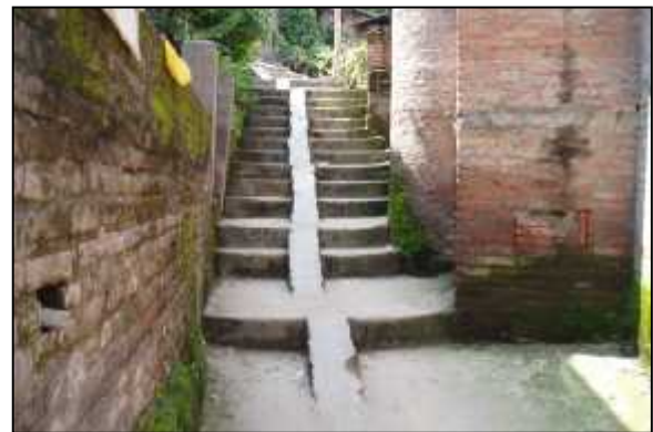
Steps to climb the settlement
