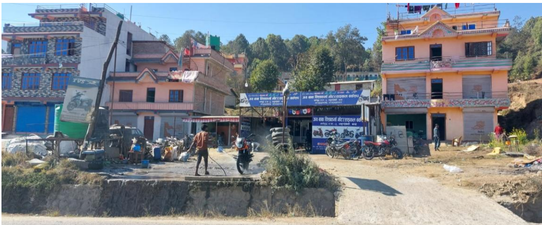
Figure 66 Modern RCC houses alongside highway
