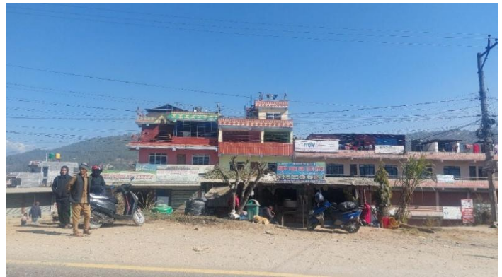
Figure 34 Structures along Road
