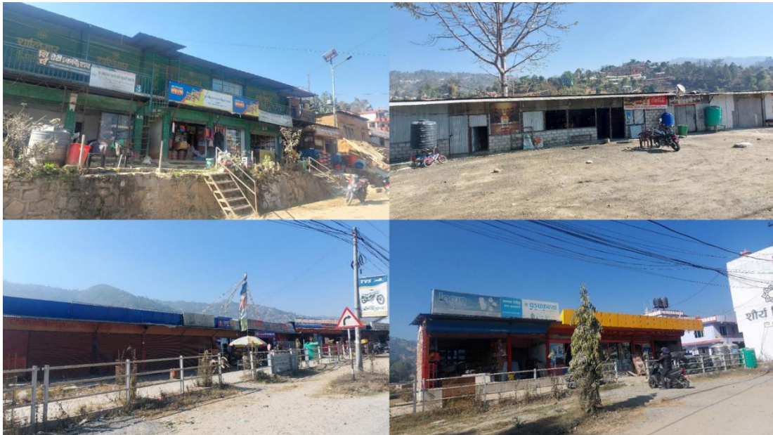
Figure 67 Temporary Structures along highway
