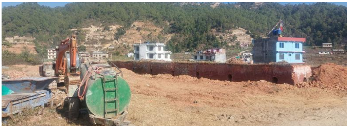
Figure 44 Condition of Brick Kilns
