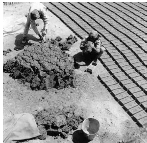
Photo 1: Making of Bricks using clay
