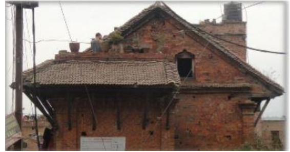
Photo 3: Traditional roof structure
