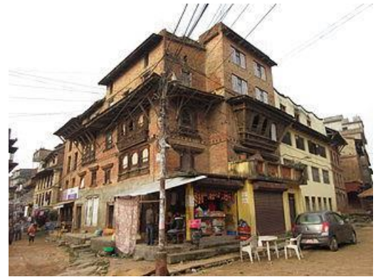
Photo 8: Traditional residential buildings of Sankharapur
