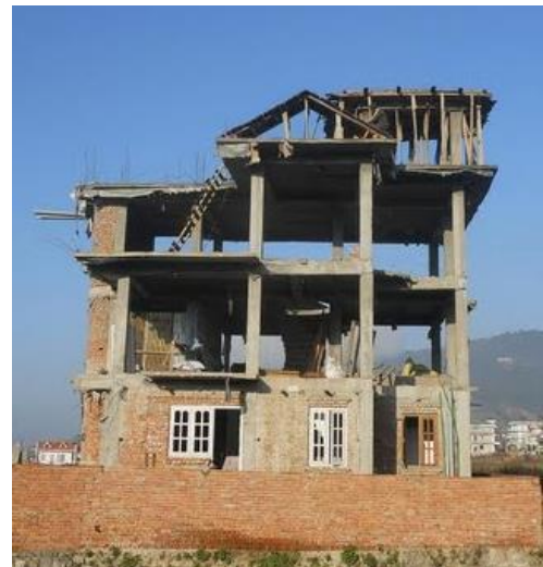
Photo 9: Modern house construction after earthquake in Sankharapur municipality
