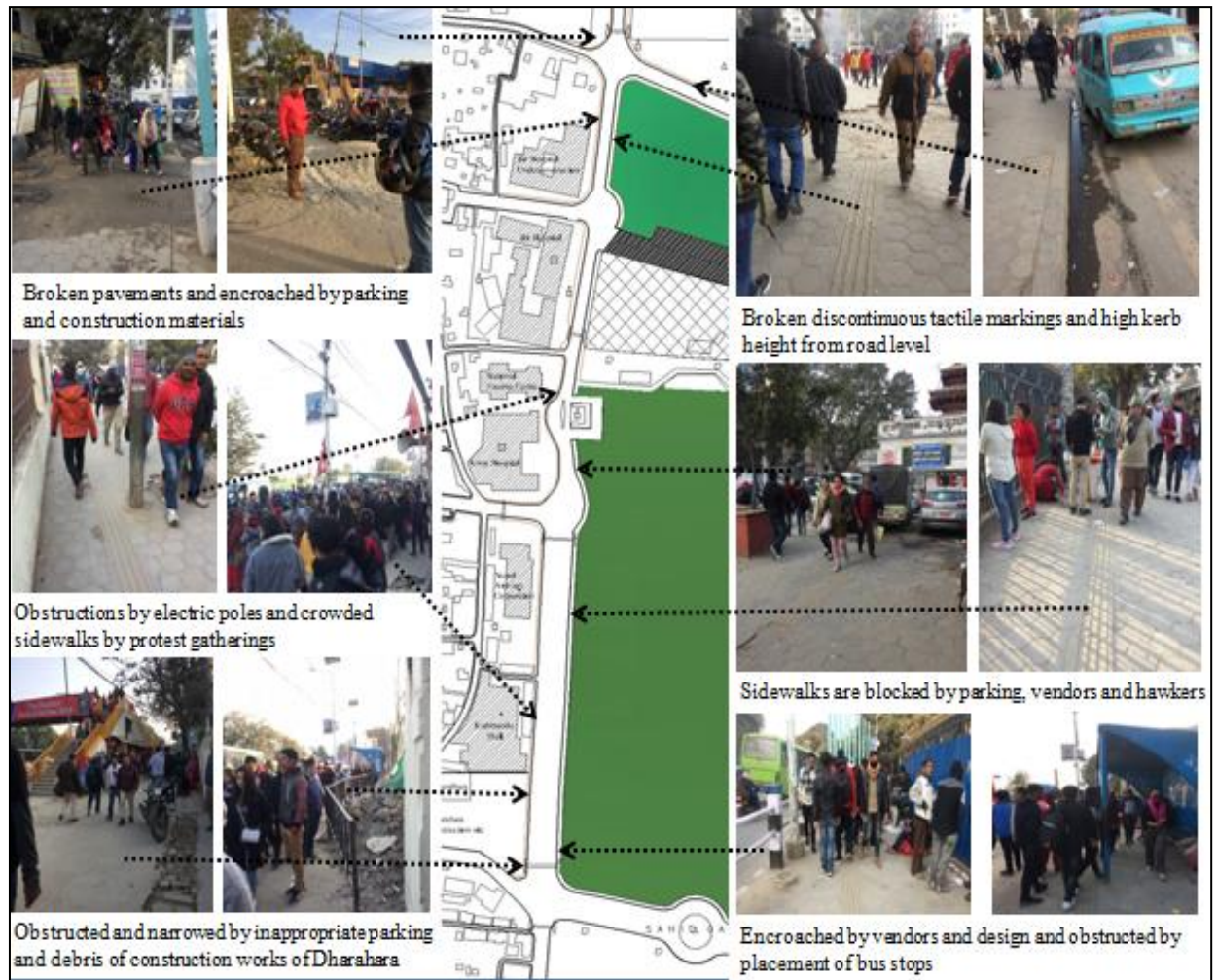
Figure 31. Obstructions in the sidewalks
