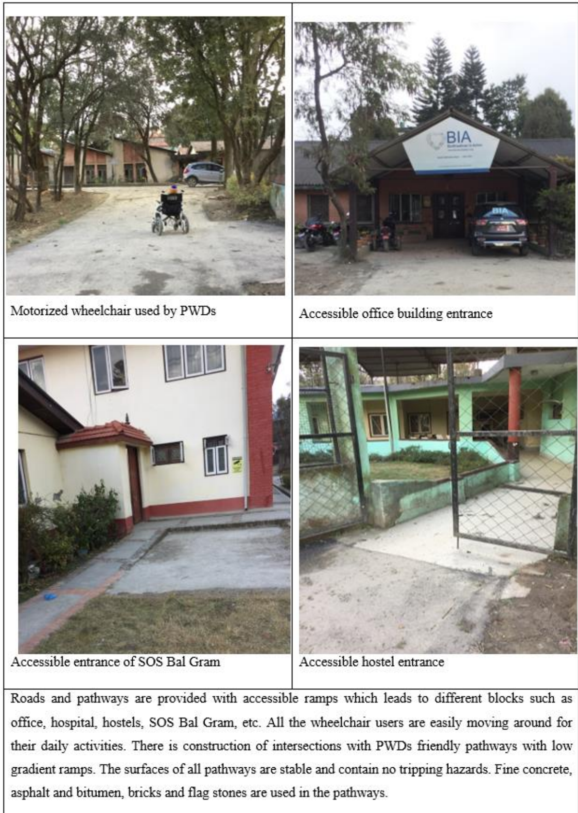
Figure 15. Examples of elements of accessibility within the premises of Khagendra Nawajeevan Kendra
