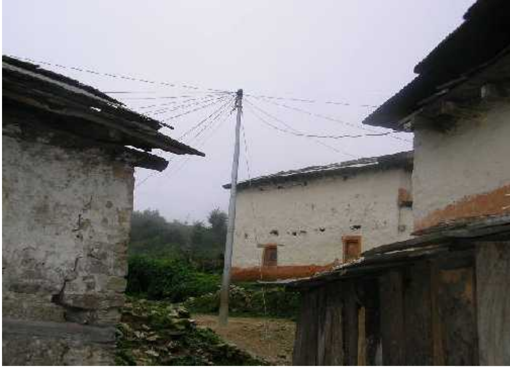
Photo 3: Web of wires! Web of Electricity Service cables in ward number 7.
