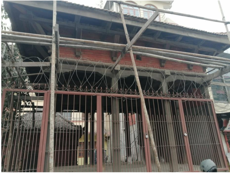
Figure 12: Sorakhutte Pati under Construction
