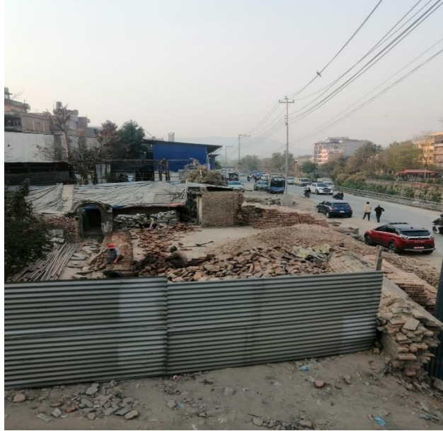
Figure 32: Rubbles of a Pati at the side of Bishnumati Bridge
