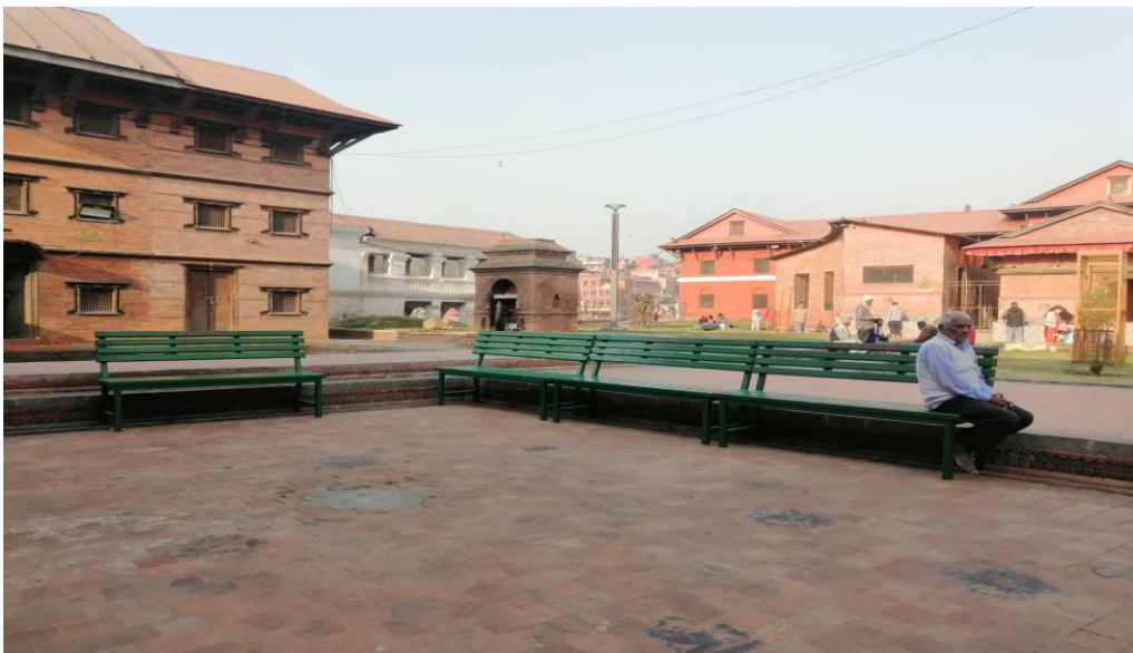
Figure 31: Area where Saptami Shraddha Sattal after demolition
