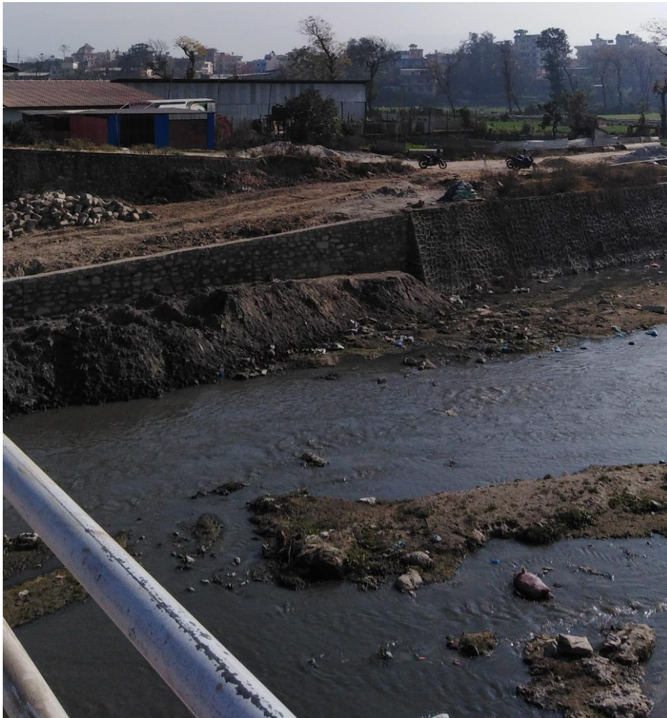
Figure 4.9 Present Condition of Manohara River and Road Construction
