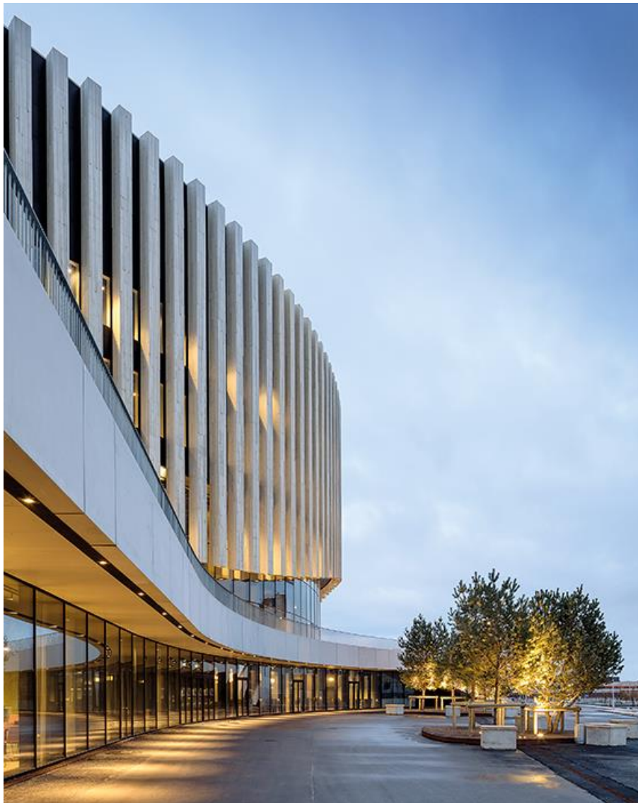
Figure 3.22 Roof Wooden Shutters in Royal Arena
