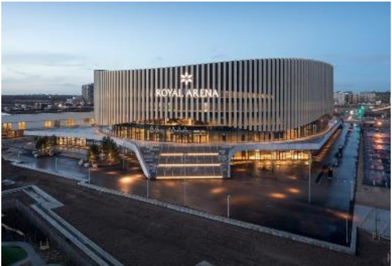
Figure 3.17 Royal Arena, Denmark
