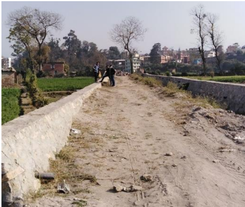
Figure 4.4 East Access Road Under Construction to Link with Ring Road
