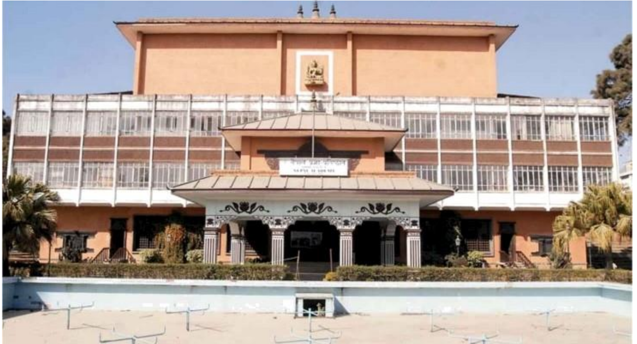
Figure 3.27 Nepal Academy Hall Front Facade
