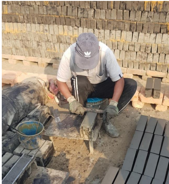
Figure 2. Fair face of brick smoothed with a knife
