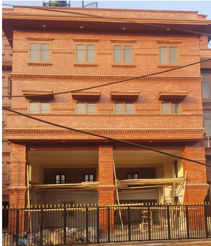
Figure 29. Newly built office building of Balaju industrial area
