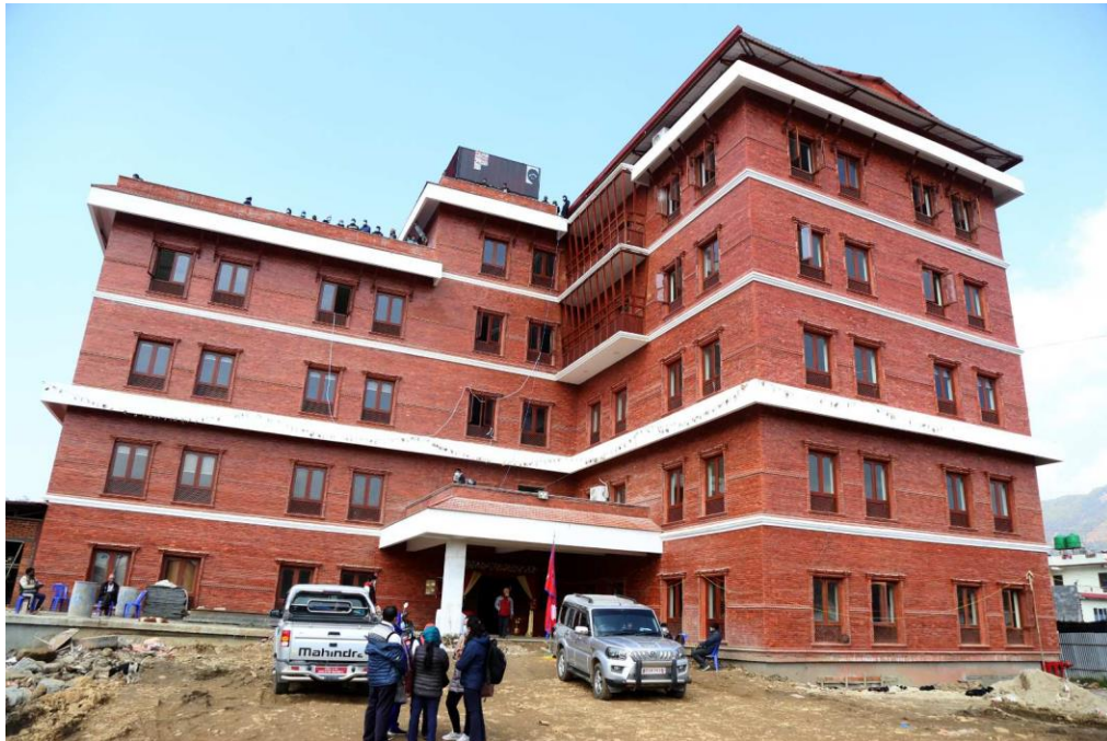
Figure 31. Newly built building of Chandragiri Municipality (Source: https://www.chandragirimun.gov.np/sites/chandragirimun.gov.np/files/field/image/viber_image_2022-02-07_20-08-22-779.jpg )
