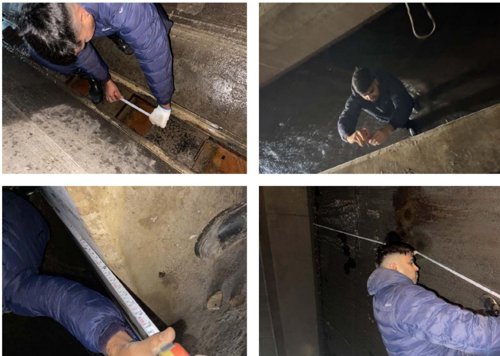
Figure 19 Measuring various Dimensions of Desander of MMHPP
