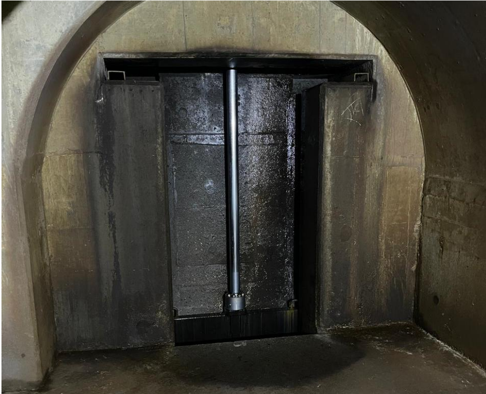
Figure 13 Flushing Gate of Desander in MMHPP
