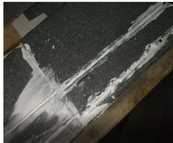
Figure 3-24: Joining wing sections using Fevicol SH
