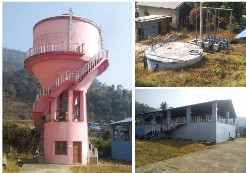
Figure 13 Existing Water Infrastructure of DWSMB
