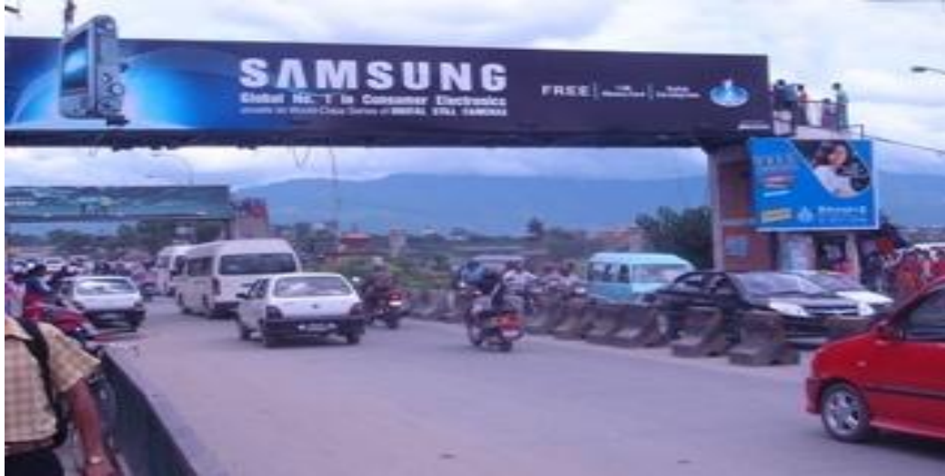
Figure 4.8 Sahid Gate Bridge: Where are the drivers supposed to look?
