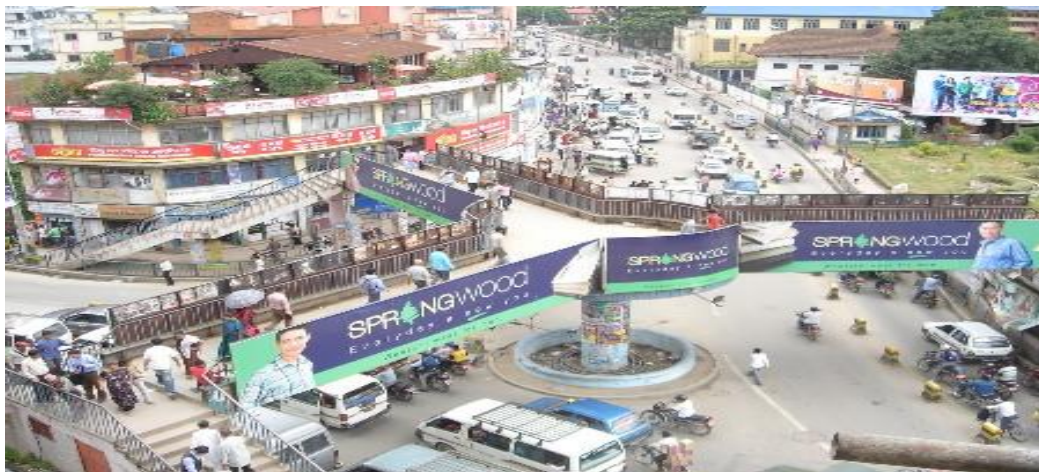
Figure 4.9 Jamal Bridge: Bird's Eye view
