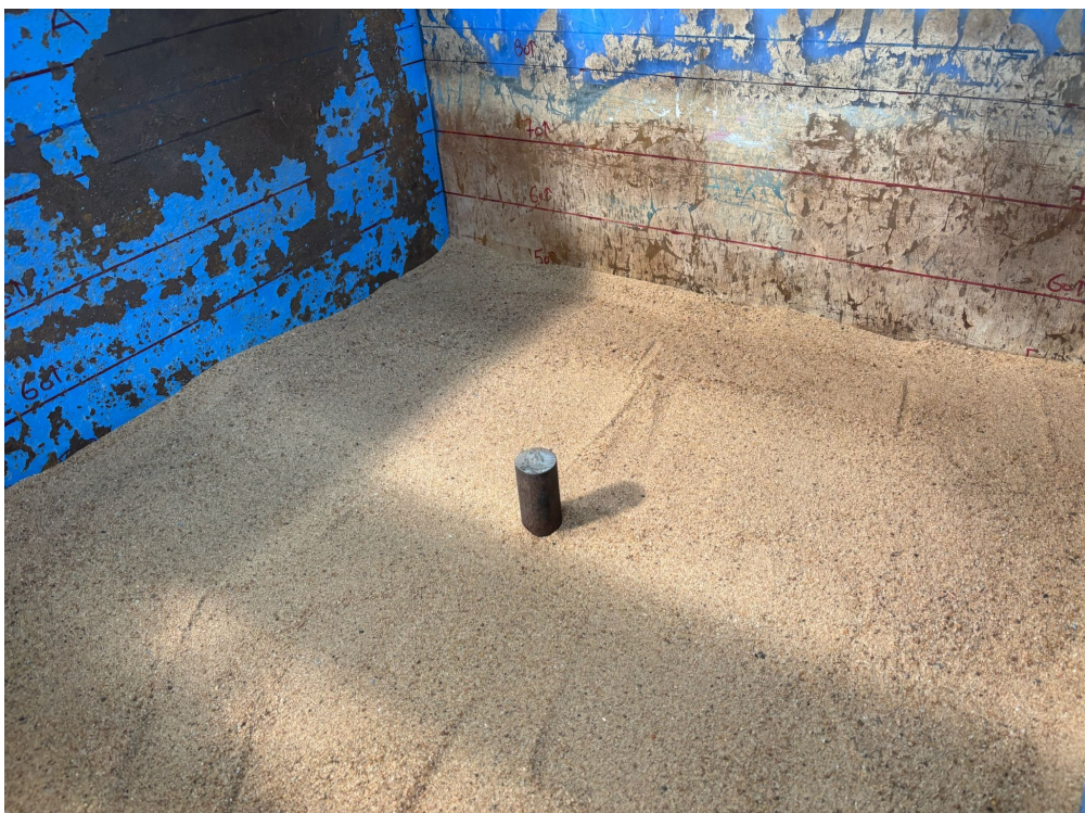
Figure B.15: Steel pile installation.
