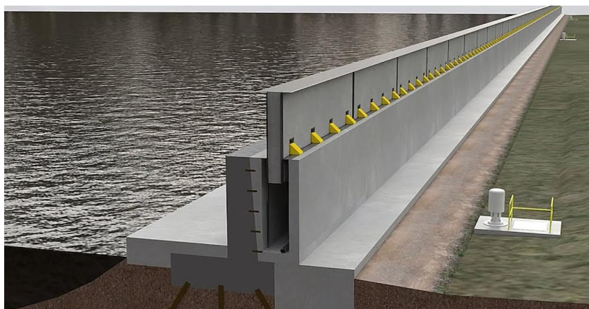
Figure 30 Temporary Flood walls
