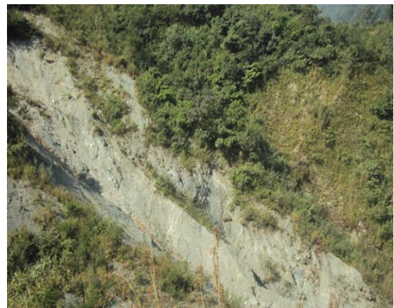
Figure 18: View of the landslide in the upper-right part
