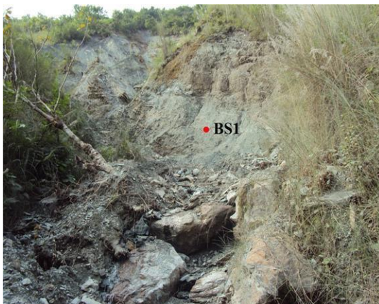
Figure 17: Sindhure Khola slide seen from road side
