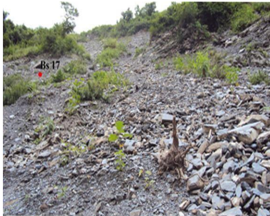
Figure 12: View of Virkuna Gaira Landslide (Ch 26+00) as seen from the highway
