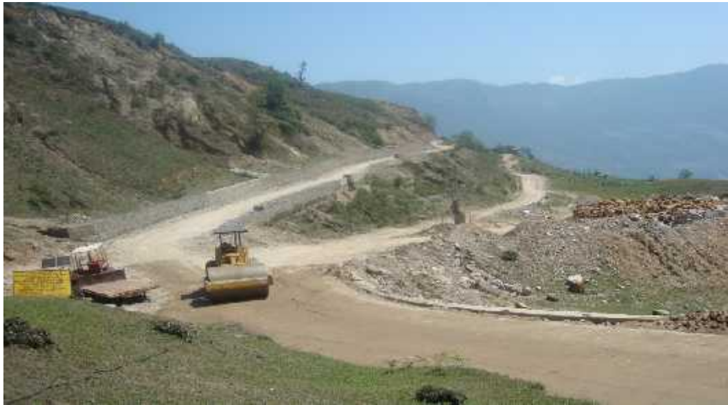
Way to TMJ and Sabhapokhari Area under Construction
