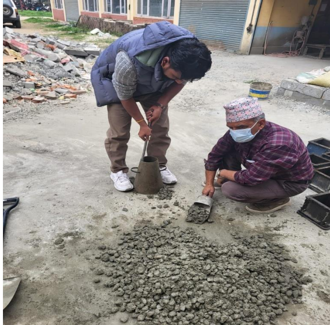
Figure 33: Slump testing for fresh concrete
