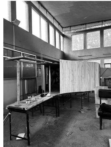
Figure C.11: Assembly of the Tunnel In progress
