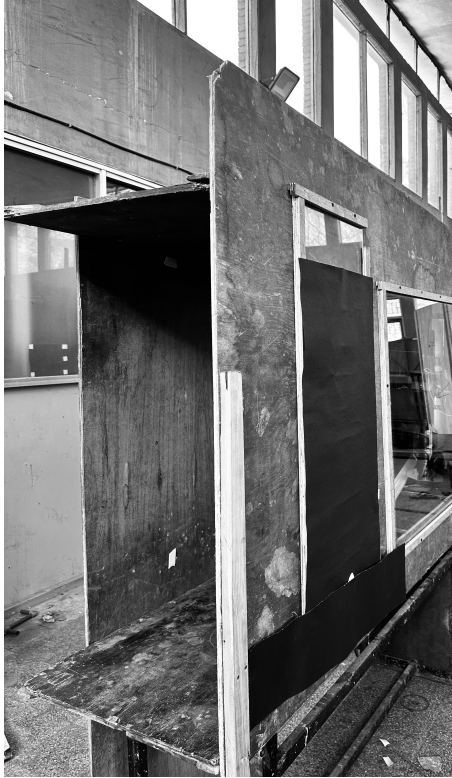
Figure C.13: Detachable Extension (520\text{mm}(W) \times 1800\text{mm}(L) \times 1000\text{mm}(H))
