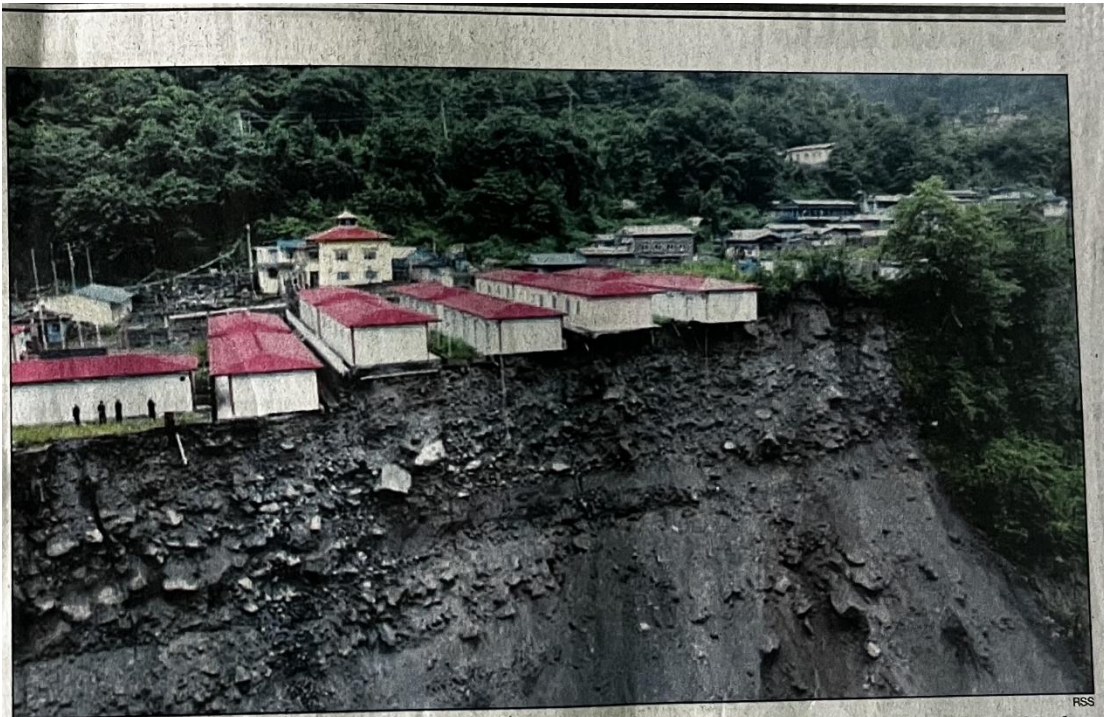
A view of endangered houses in the settlement of Danaque of Naso Rural Municipality of Manang due to flood in the Marsyangdi River, on Friday.
