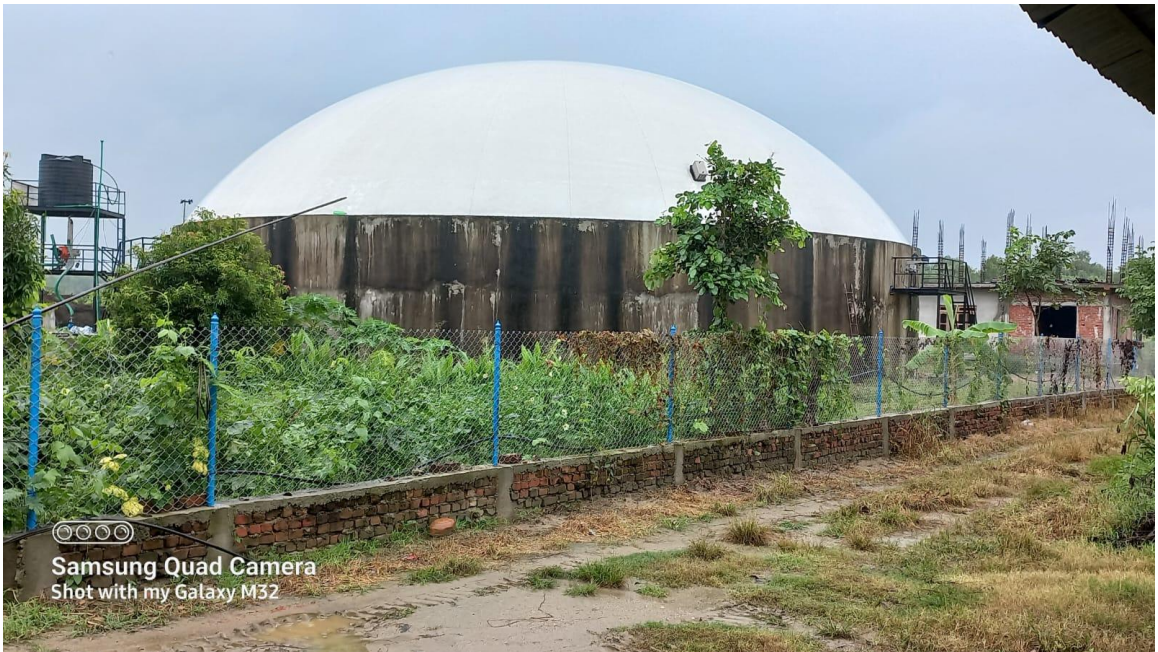
Annex 2: Outer View of Biogas Plants
