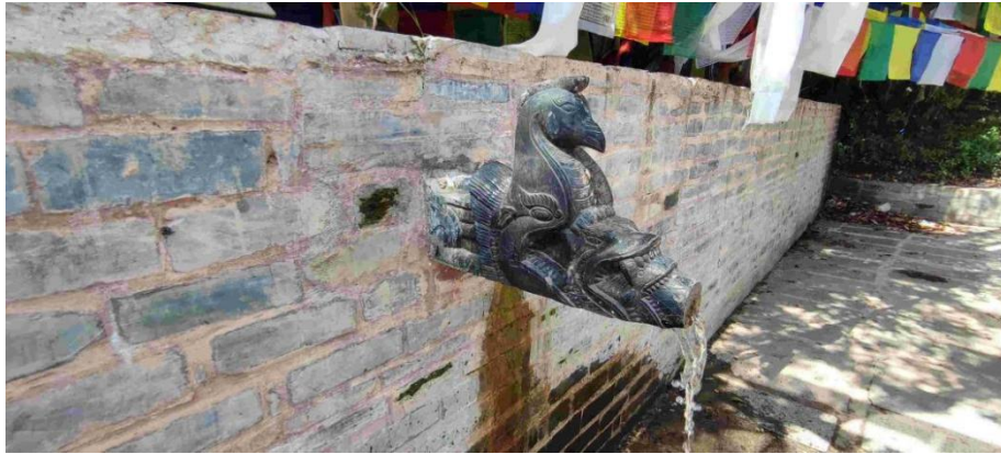
Figure 20: Photo of Water Conduit
