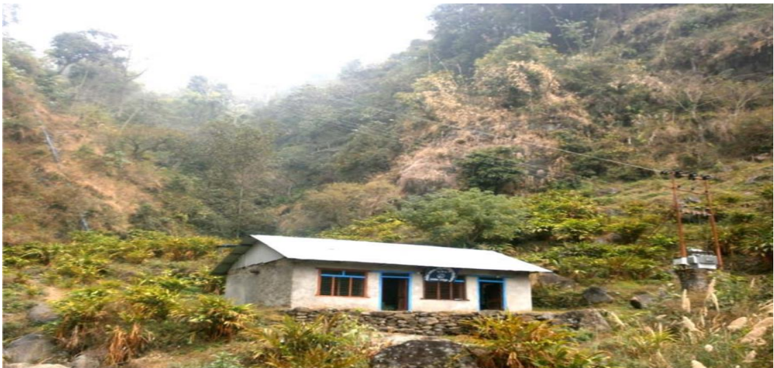
Figure 35: Powerhouse of Methem Khola MHP (District Development Committee, Taplejung, 2016)
