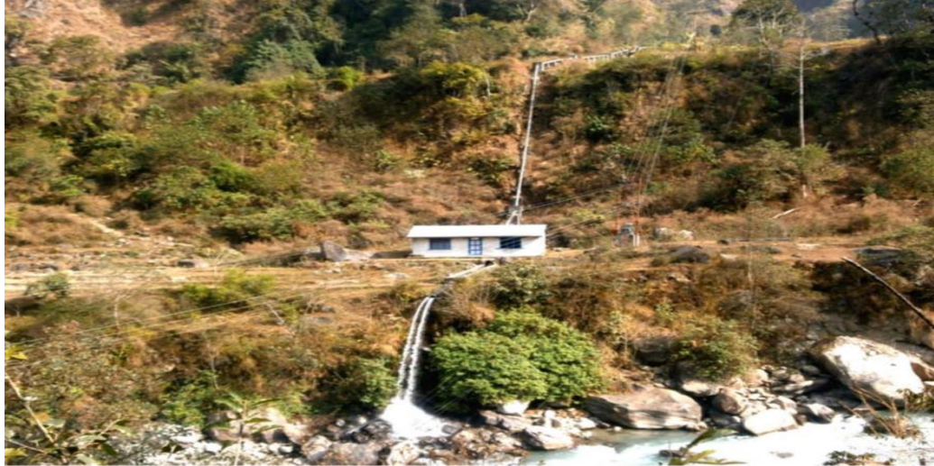
Figure 36: Powerhouse of Tewa-Mekwa Khola MHP (District Development Committee, Taplejung, 2016)
