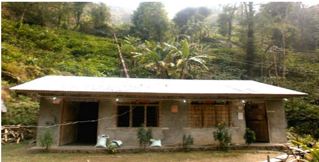
Figure 33: Powerhouse of Yafre - Mauwa Khola MHP (District Development Committee, Taplejung, 2016)
