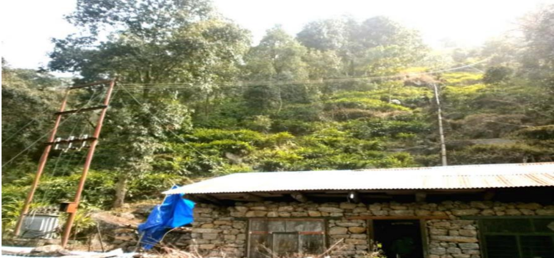
Figure 34: Power House of Tawa Khola MHP (District Development Committee, Taplejung, 2016)
