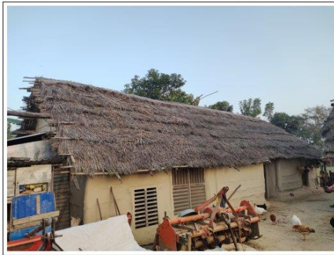
Figure 4: Case Study Building
