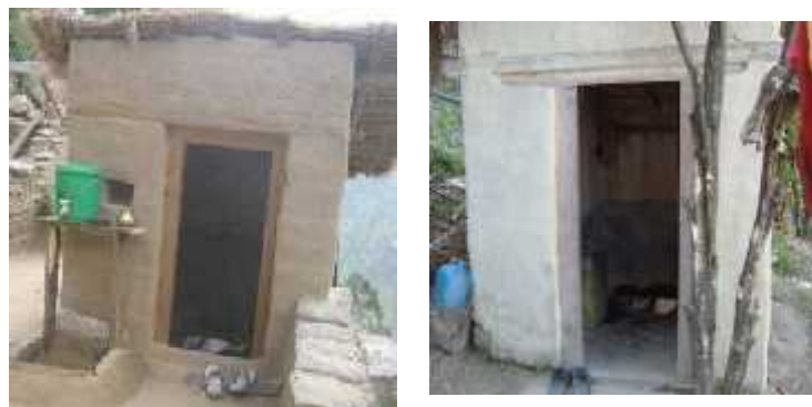
Picture -9, Toilets , constructed totally from local material (Grass Roof and mud plaster)
