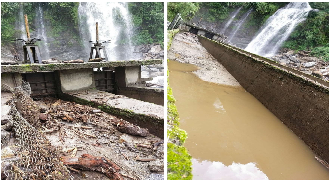
Figure 4.9: Impact of Debris Flow at Intake
