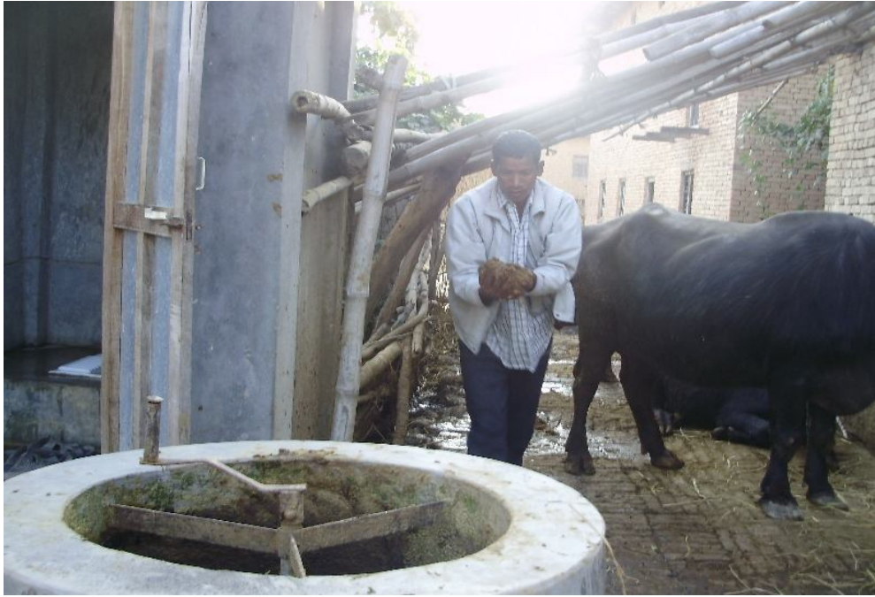
5. Mixing dung in biogas plant by users
