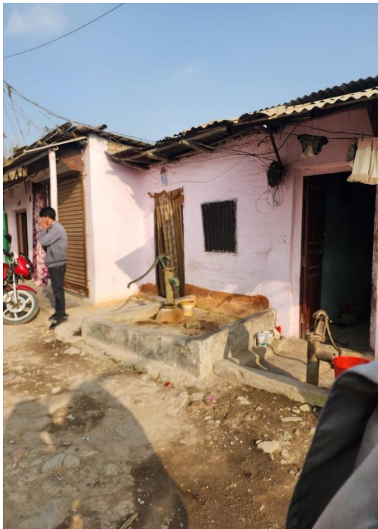
Figure 10 Jagritinagar Informal settlement: Presence of water taps in individual houses
