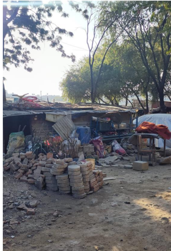
Figure 13 House construction in Thapathali informal settlement
