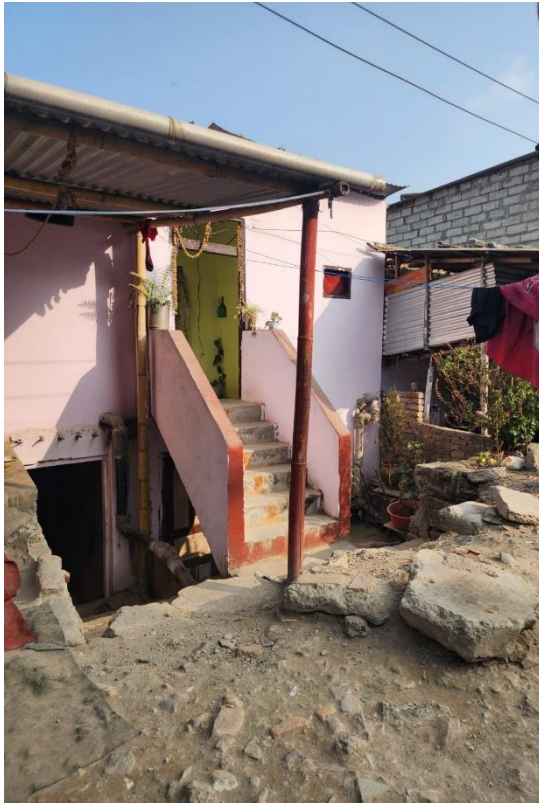
Figure 12 House construction in Jagritinagar informal settlement
