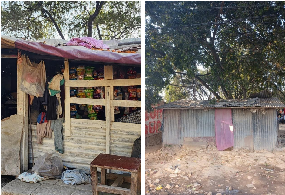
Figure 8 Residence construction in Thapathali Informal Settlement
