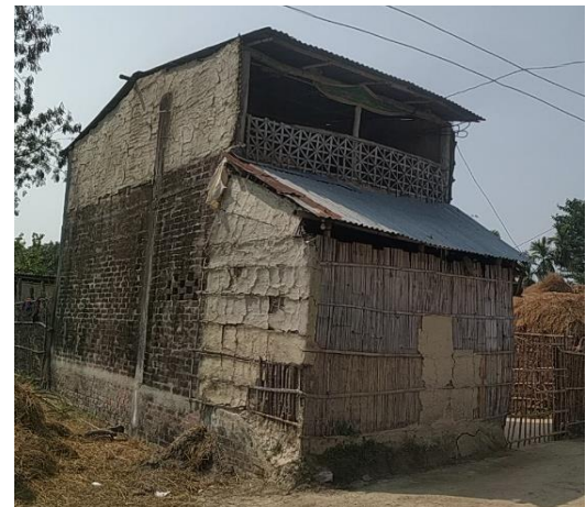
Figure 31: Combination of brick with cement; bamboo with mud as outer wall
