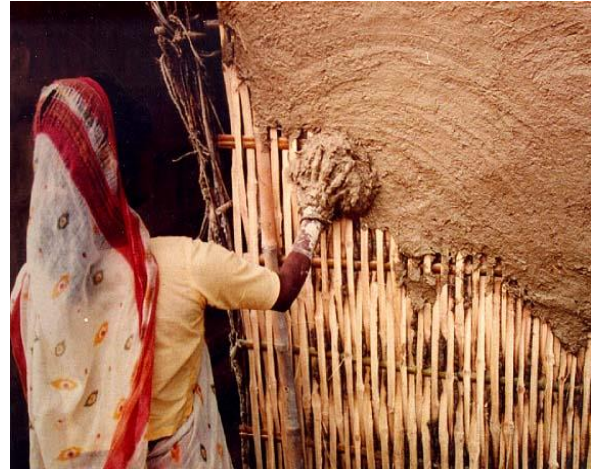
Figure 28: Building and shaning a wall: first.
