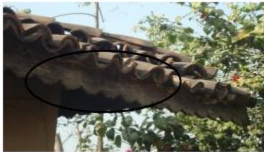
Figure 26: Detailing of clay tiles (khapda) at roof
