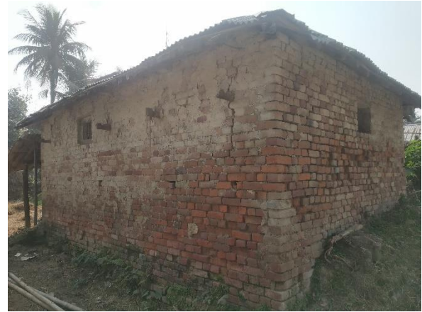
Figure 34: Brick and mud mortar in outer wall
