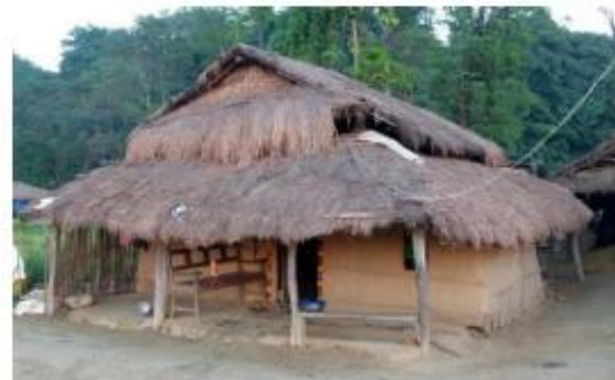
Figure 36: Tharu home in Chitwan with a large roof overhang and a covered veranda
