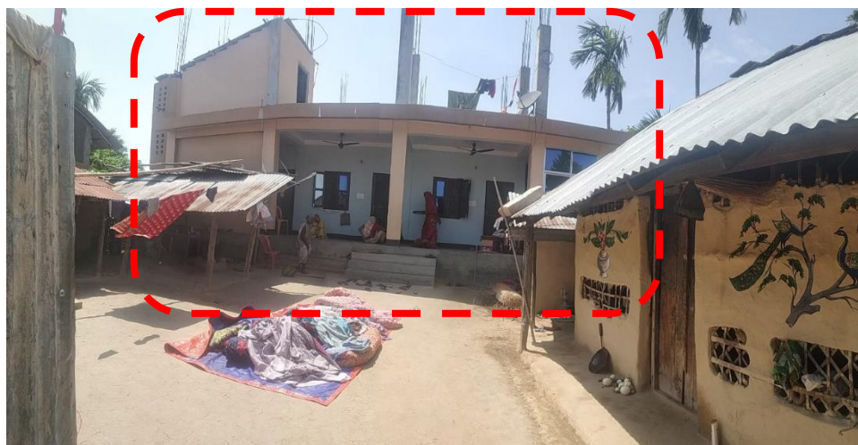
Figure 117: Replacement of mud house into RCC house; Residence of Ram Subaran Chaudhary after transformation
