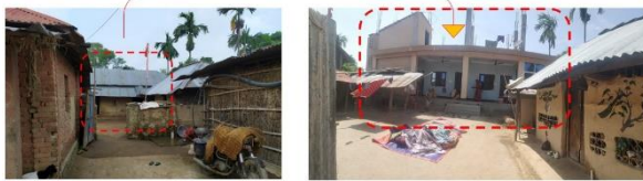
Fig: Replacement of mud house into RCC house; Residence of Mr. Ram Subaran Chaudhary after transformation
