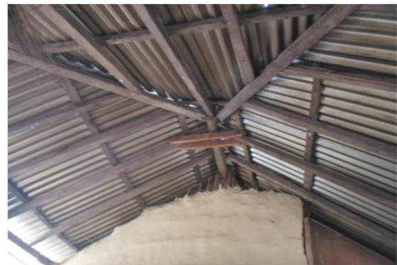
Figure 27: Joint detail of beam and post
