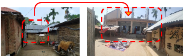
Figure 6: Replacement of mud house into RCC house; Residence of Mr. Ram Subaran Chaudhary after transformation
