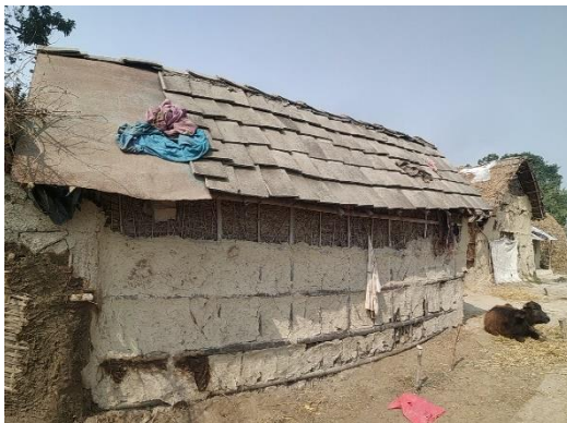
Figure 41: Different types of cement tiles used on roof
