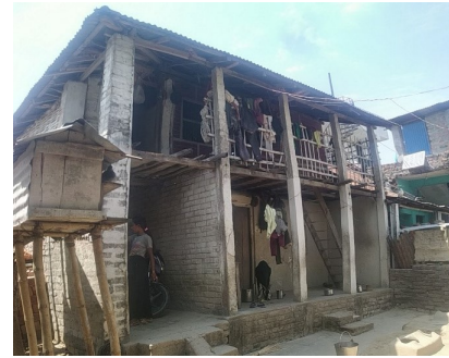
Figure 7: Addition of pillar and concrete block in old mud structure; Residence of Mr. Raj Kumar Chaudhary
