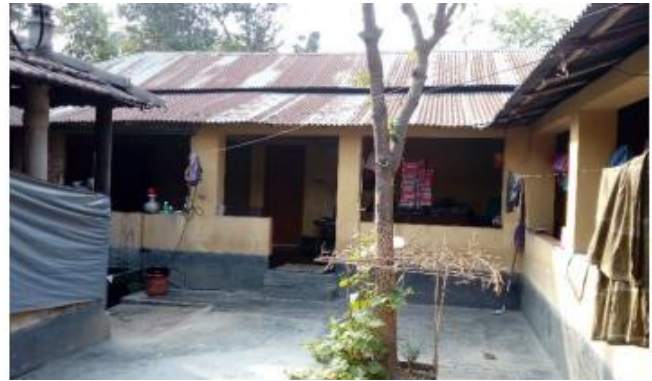
Figure 69: The inner courtyard is covered by cement-plaster to make it clay free during rain
