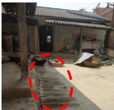
Figure 154: Use of broken tiles on ground for rain water drainage
