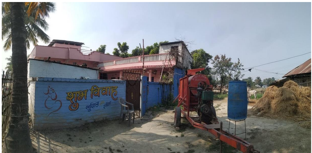
Figure 164: View from street of house on. 7
