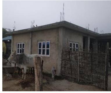
Figure 148: View from street
