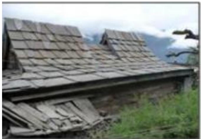
Figure 48: Steep Pitched roof
