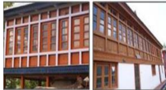
Figure 50: Transformed verandah with use of glass
