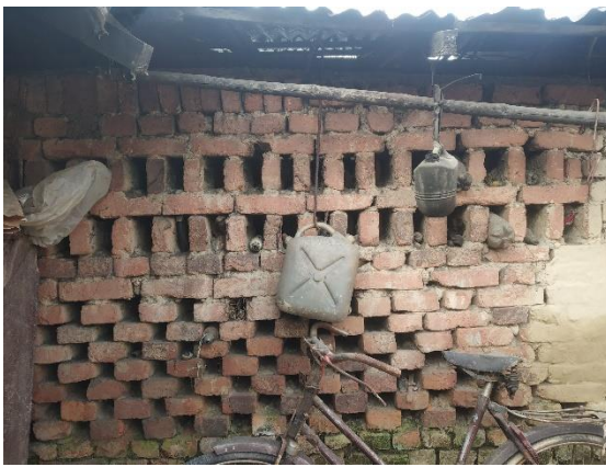
Figure 33: Brick pattern for ventilation
