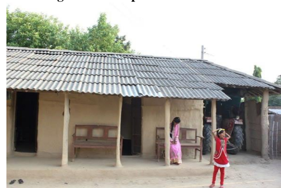
Figure 41: Different types of cement tiles used on roof
