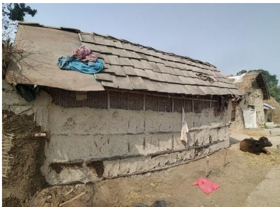
Figure 106: Bamboo strips with paddy straw and mud plastered wall
