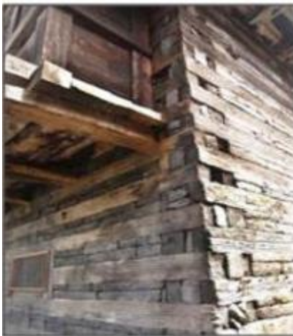
Figure 49: Kath and Kunal construction
