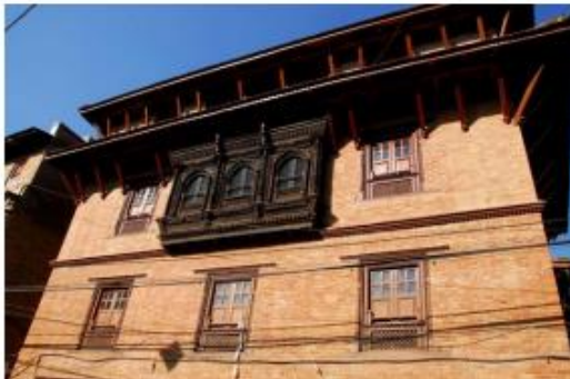
Figure 6: Façade of Newar house with big wood carved window and large roof overhang
