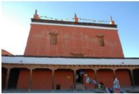
Figure 7: Typical Small windows in building façade in Upper Mustang
