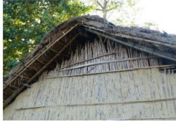
Figure 37: Gable opening for air circulation in Tharu House, Chitwan
