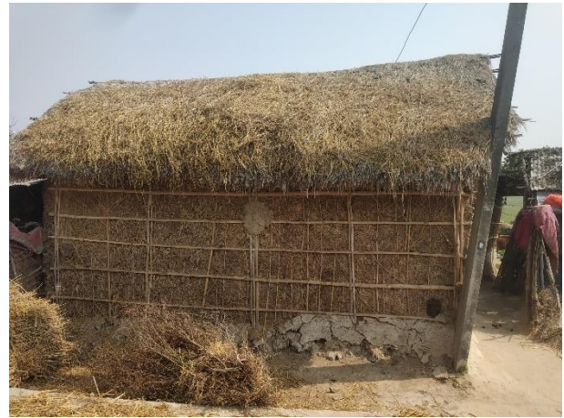
Figure 32: Use of nigalo bamboo, bamboo leaves, straw and mud as outer wall
