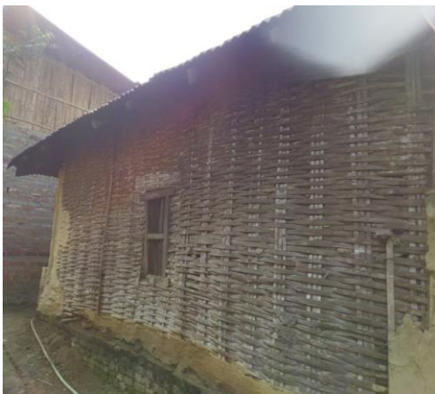
Figure 33: Use of bamboo strips and mud in wall
