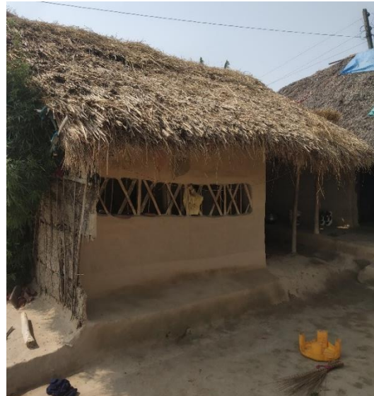
Figure 104: Kitchen with horizontal window for proper ventilation
