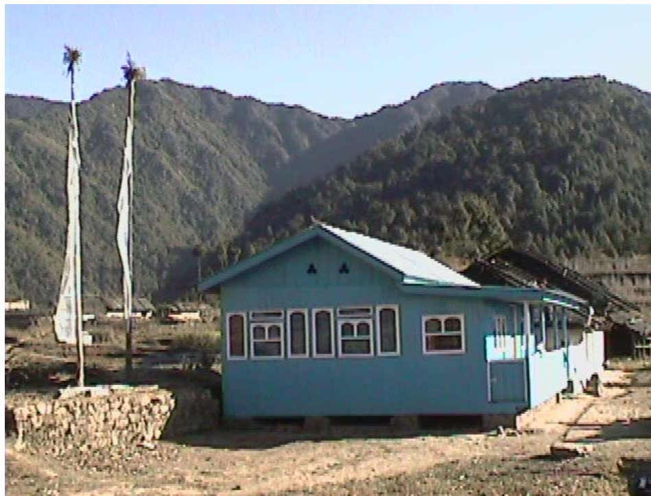
Figure 30. New Hageham Home . Prem Tamang's newly constructed home in Hageham. It is made of 2x4 planks and covered with corrugated tin painted blue. Kaiyakatta lies tucked in the pass far in the background.
