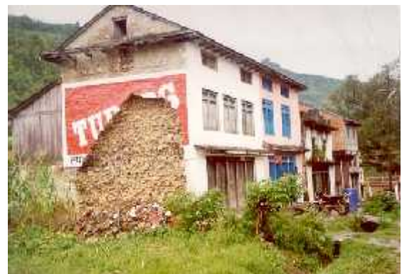
Earthquake in Dhading 2045 BS
