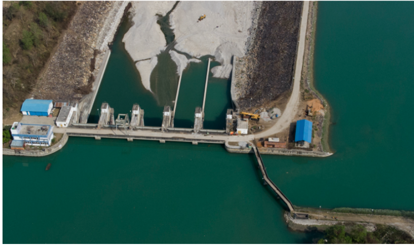
Figure 3.9: Lower Marsyangdi, hydro-power plant dam site, Aanbukhaireni
