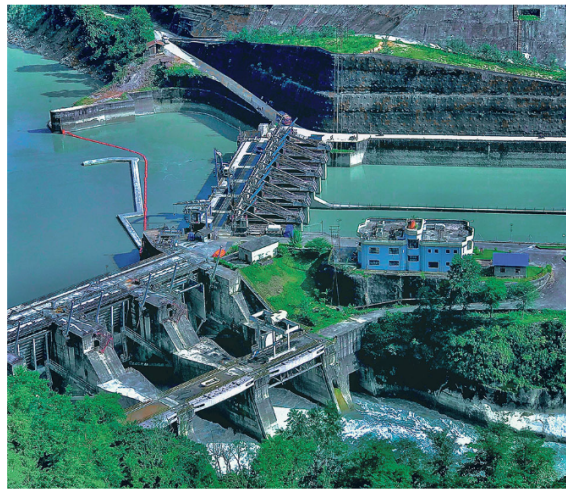
Figure 3.4: The dam, intake (bottom), spillway (top), Kaligandaki 'A' hydro-power plant
