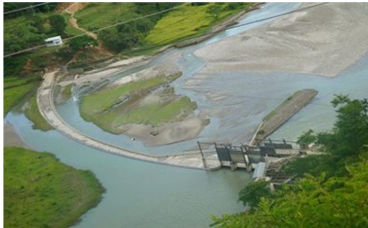
Figure 3.2: Aerial view of the catchment and dam area of Jhimruk hydropower plant
