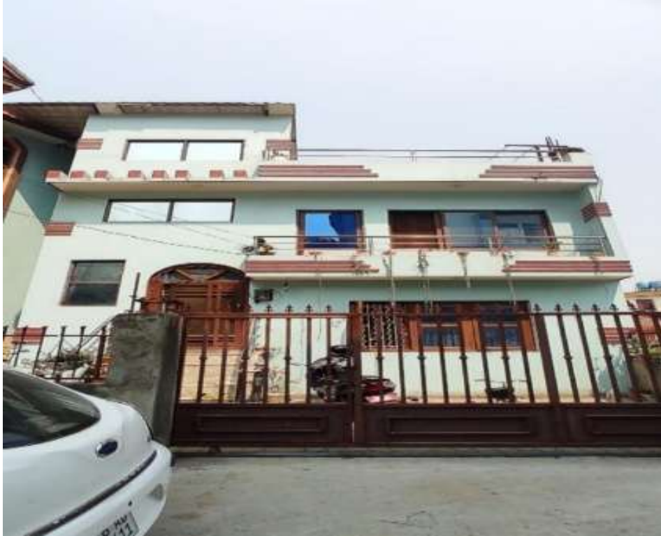
Figure 7 RCC building Maitrinagar
