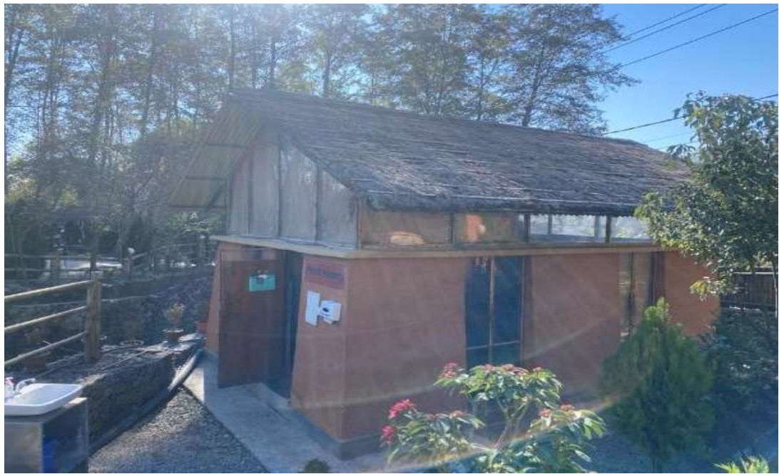
Figure 3 Dekaido Onsen for collection of indoor and outdoor temperature
