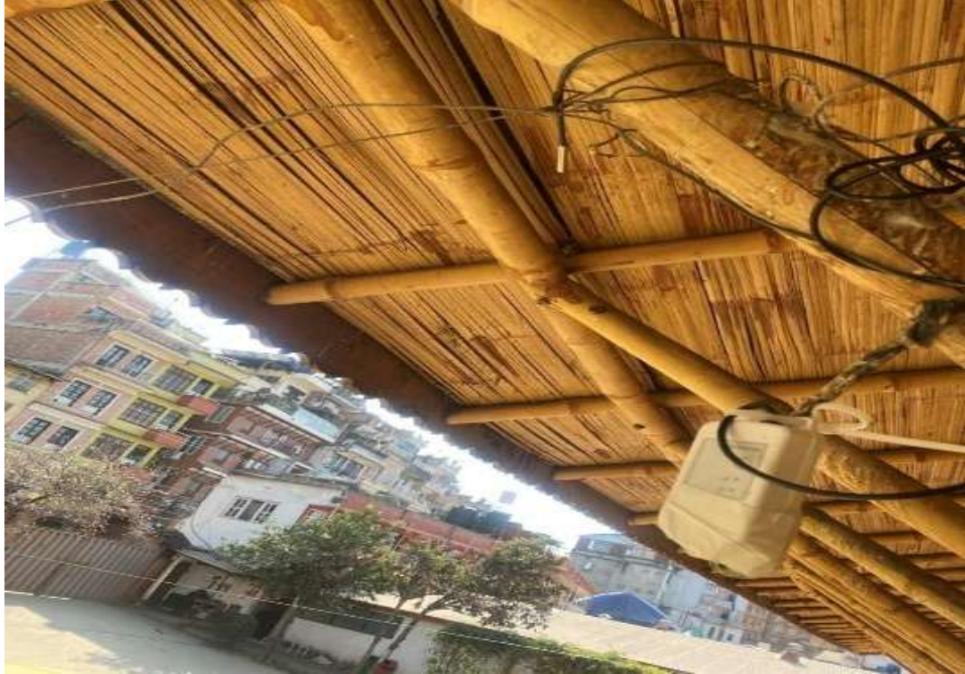
Figure 11 Hobo data logger for recording outer temperature at Madan Pustakalaya
