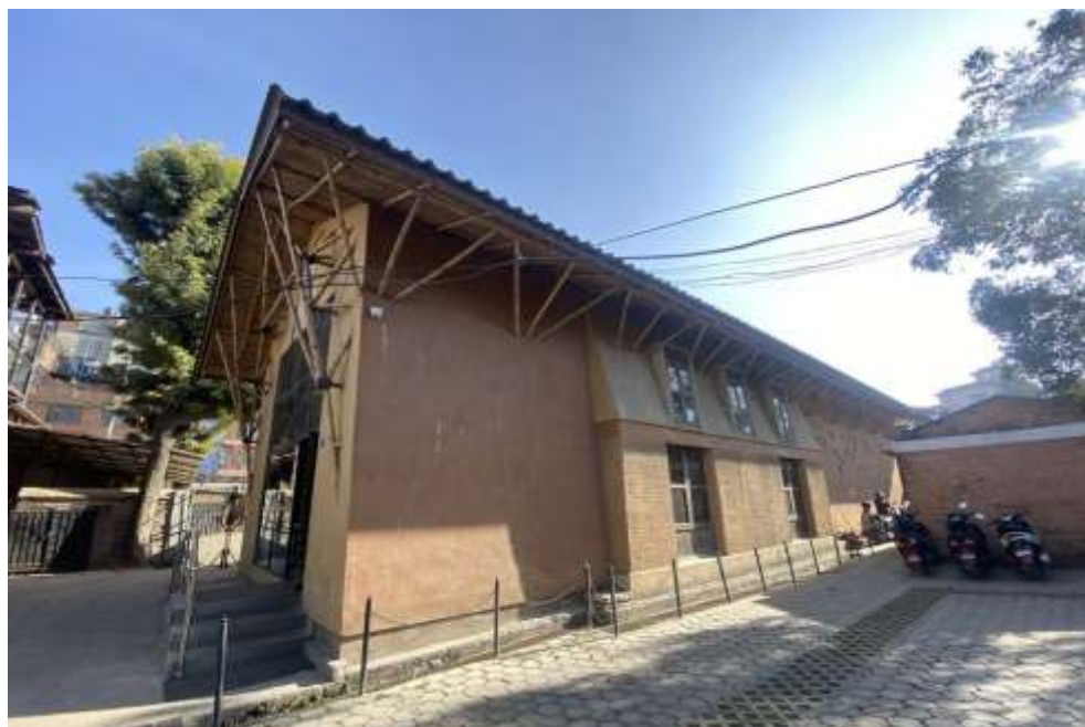
Figure 5 Madan Pustakalaya for collection of indoor and outdoor temperature
