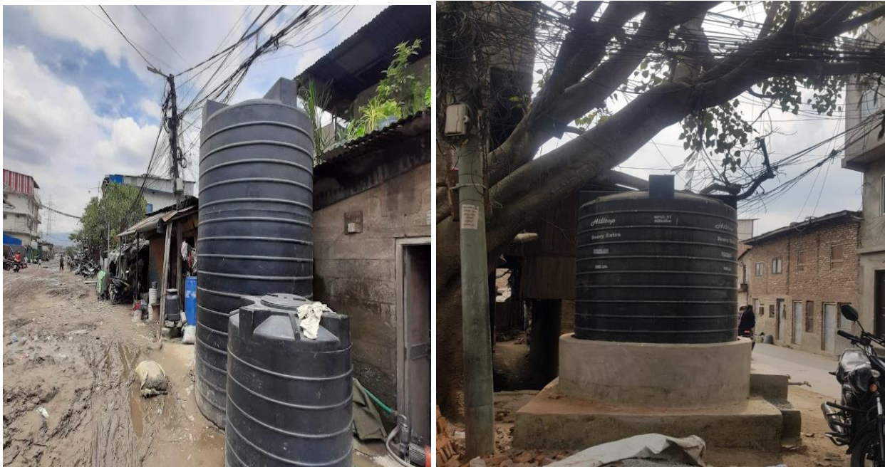
Figure 22 Water storage tank in Jagriti Nagar and Bansighat
