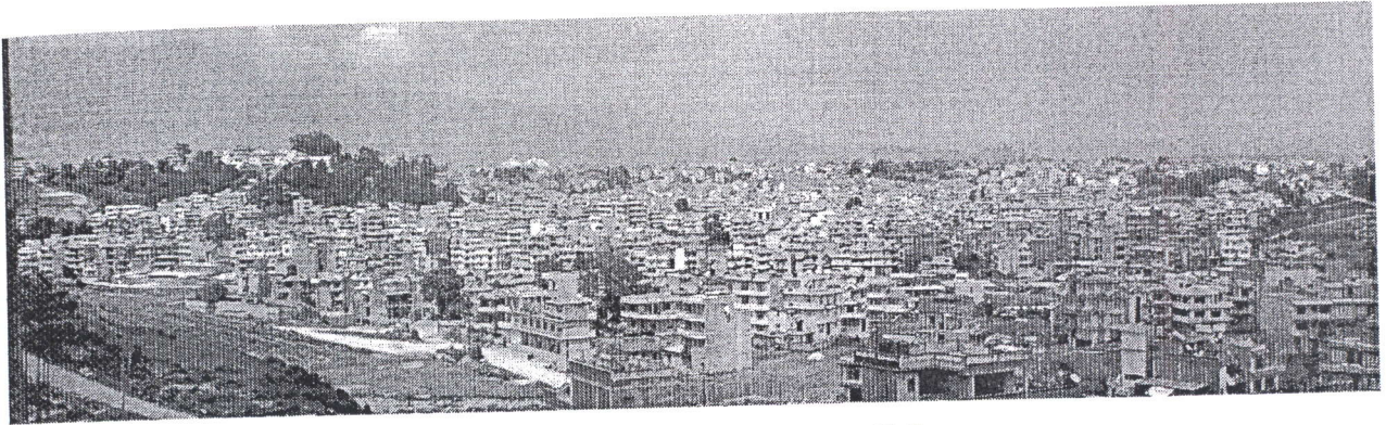
Figure 1: A perspective view of urban fringe development in Kathmandu Valley Source: Author
