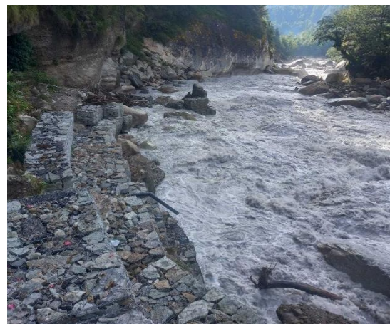
Figure 93 Embankment at the Edge of Marshyangdi River
