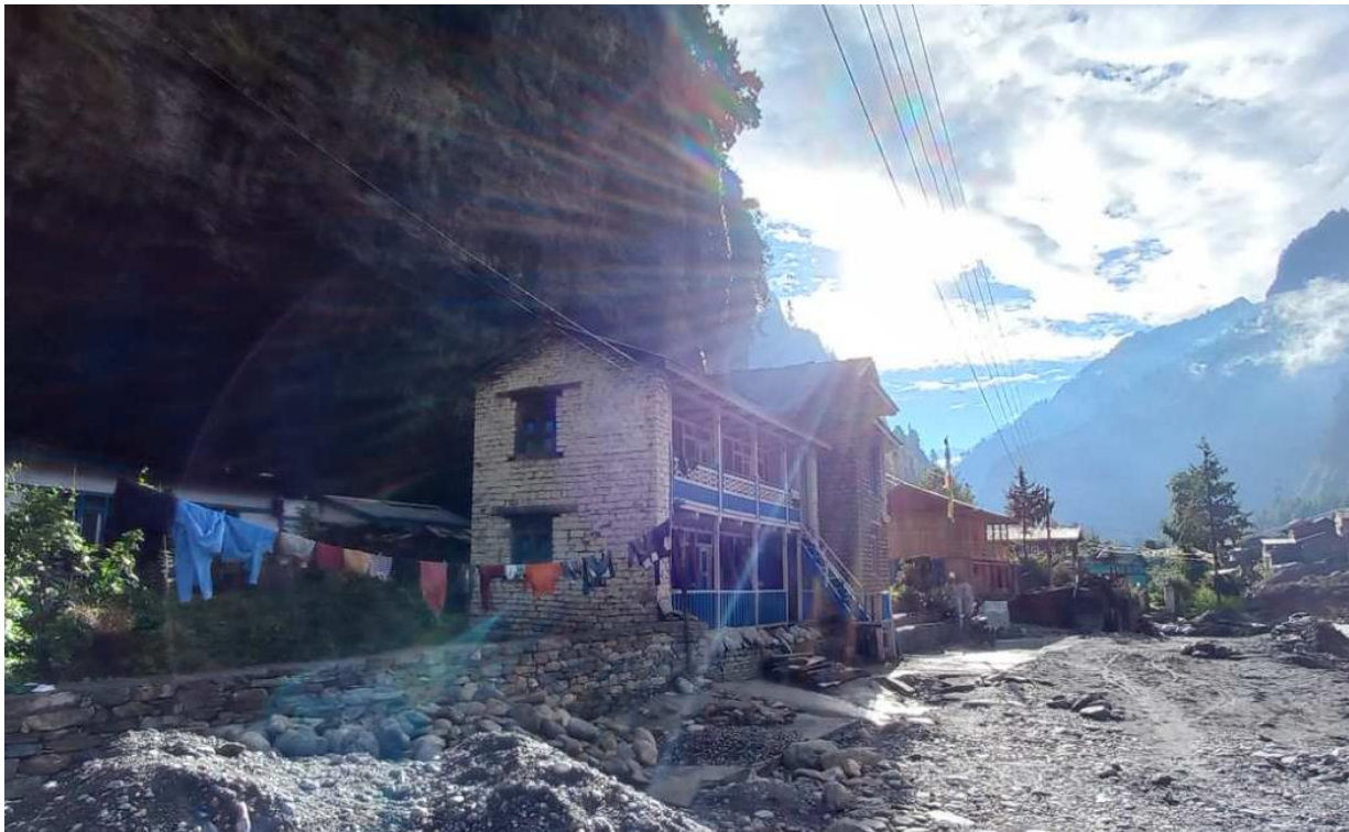
Figure 83 A local two storey house in chame with loadbearing features, traditional windows, lime plaster.
