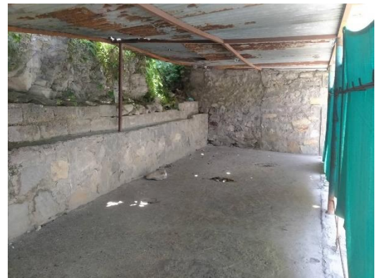
Figure 61 Common Changing Area
