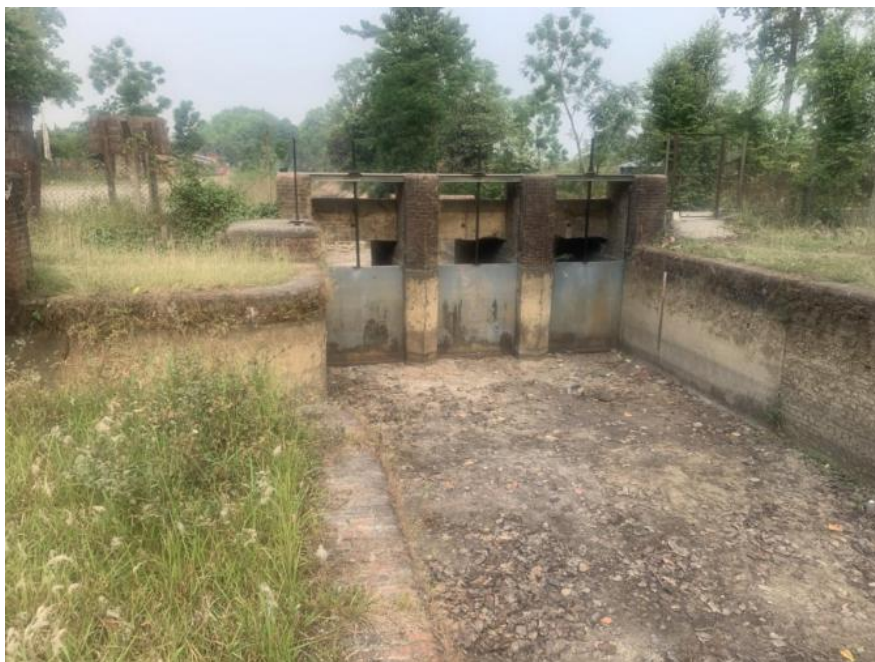
Existing condition of canal sluice gate
