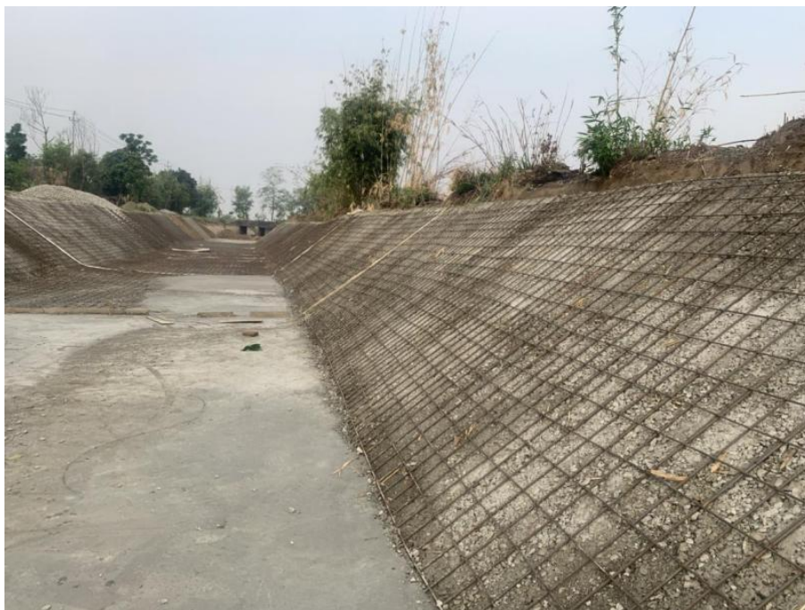
Main canal lining work at KIP
