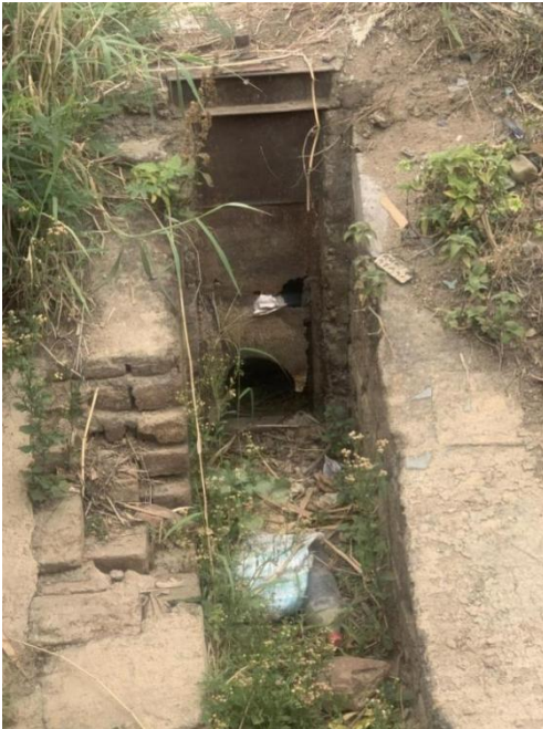
Existing canal and gate condition of KIP
