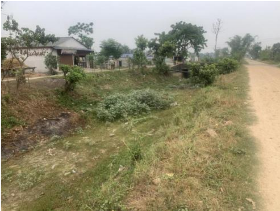
Current condition of weeding, siltation, and pollution inside Khageri irrigation canal
