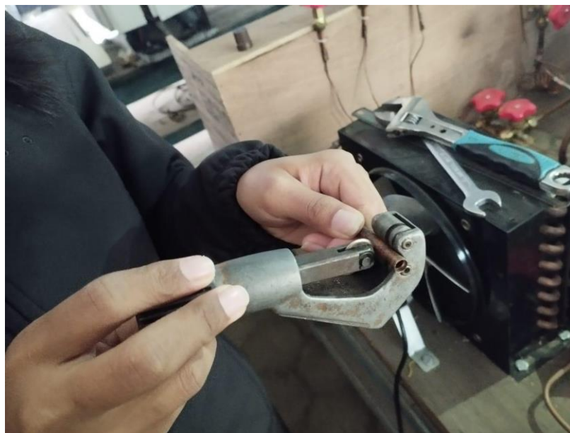
Fig: Cutting copper pipe with tube cutter
