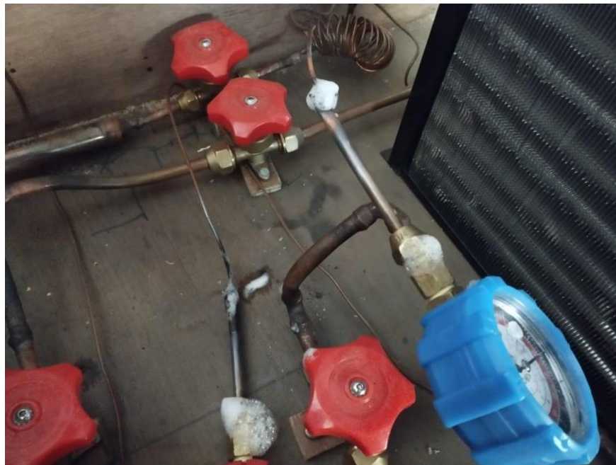
Fig: Bubble Testing
