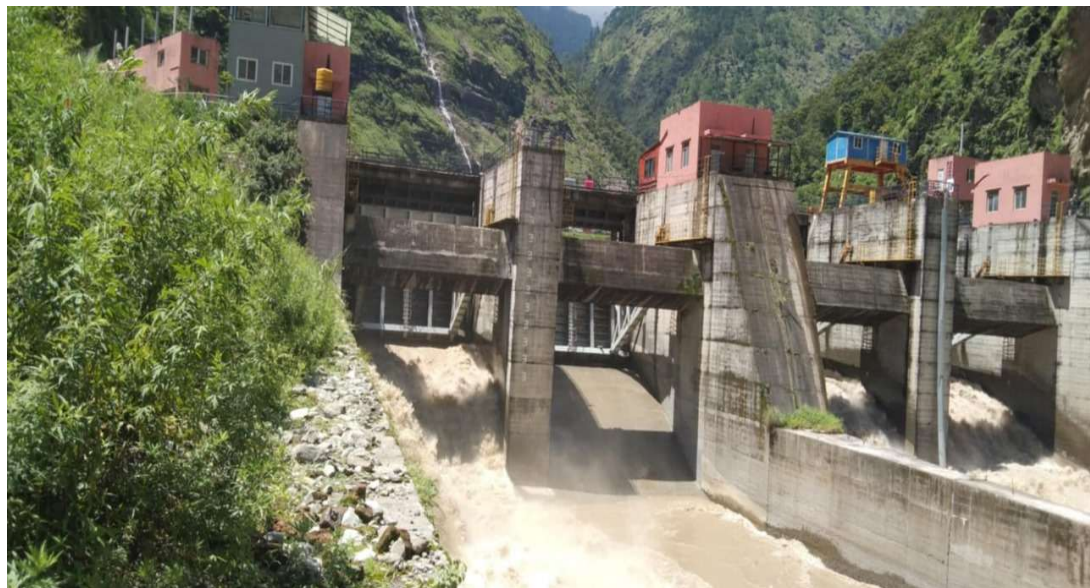
Figure 3-3: UT3A Hydropower Intake
