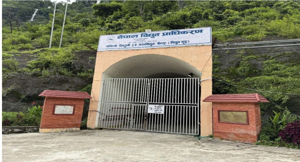
Figure 3-2: Powerhouse entrance of UT3A Hydropower Station
