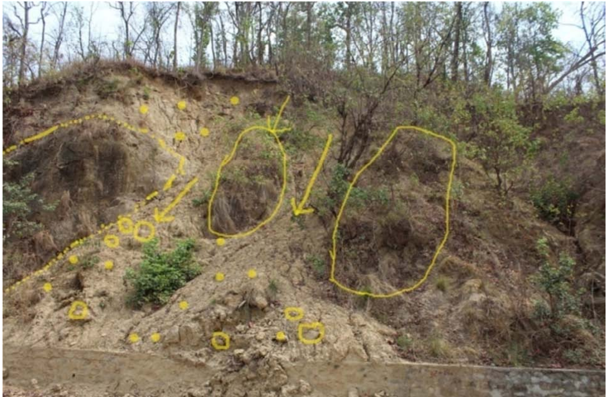
Figure 11. Landslide in conglomerate observed near Babai Bridge at Babai Valley, Surkhet.
