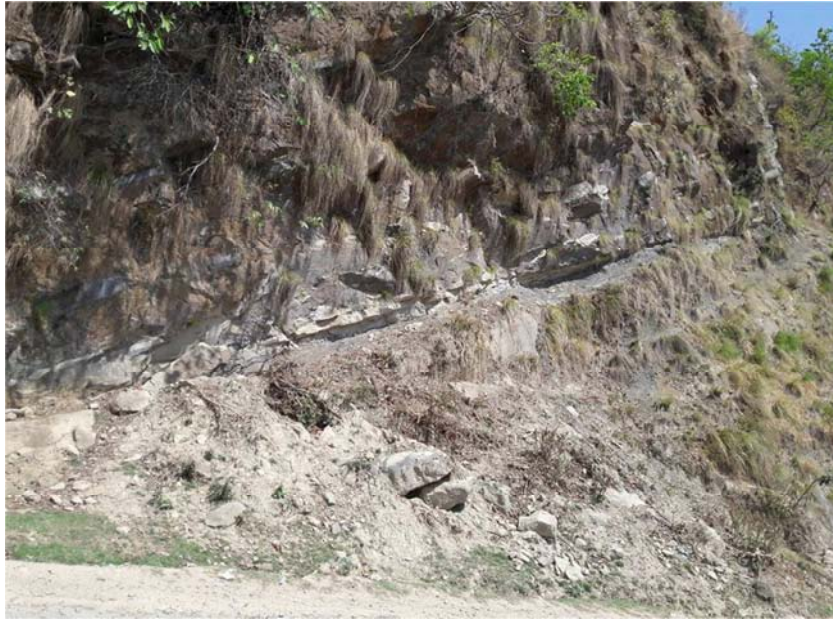
Figure 4. Exposure of Middle Siwaliks at Harre of Surkhet, along the road section.
