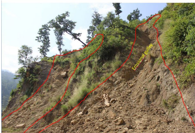
Fig. 16 Landslide caused by weathered mudstone in between the alternate layer of Mudstone and Sandstone of Lower Siwaliks (Photo taken at Upper Damdawali of Salyan district)
