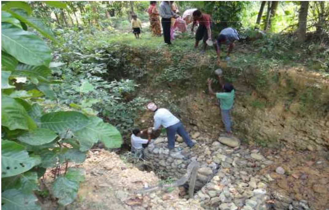
Check dam construction by CFUG Members
