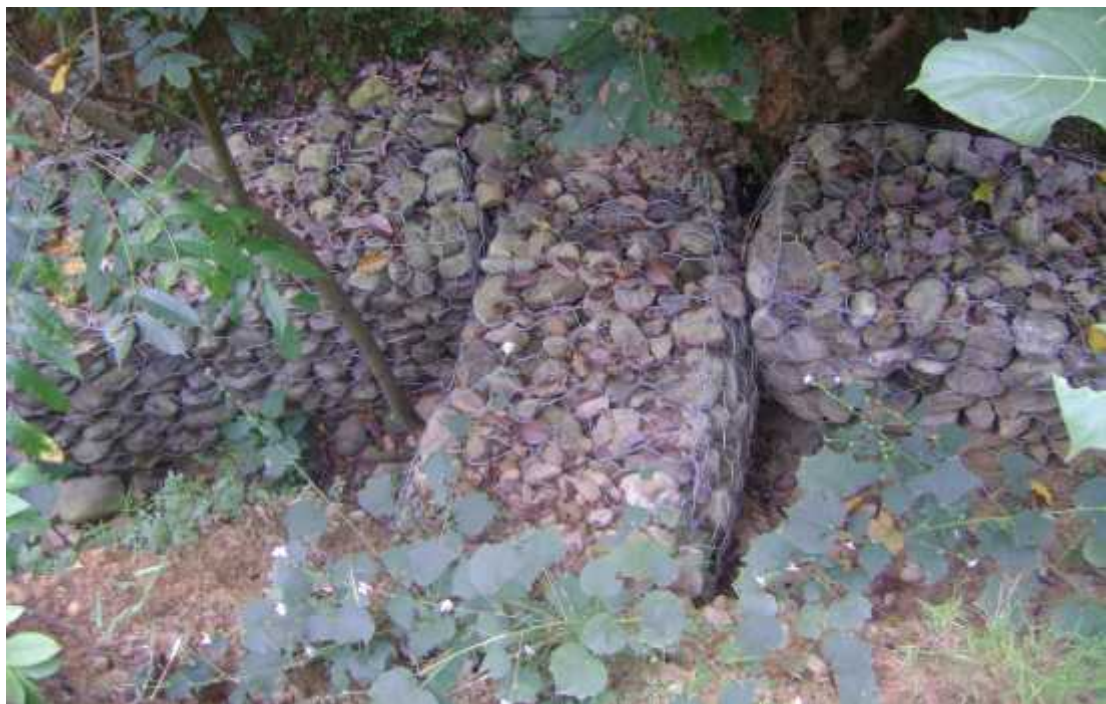
Complete check dam construction.
