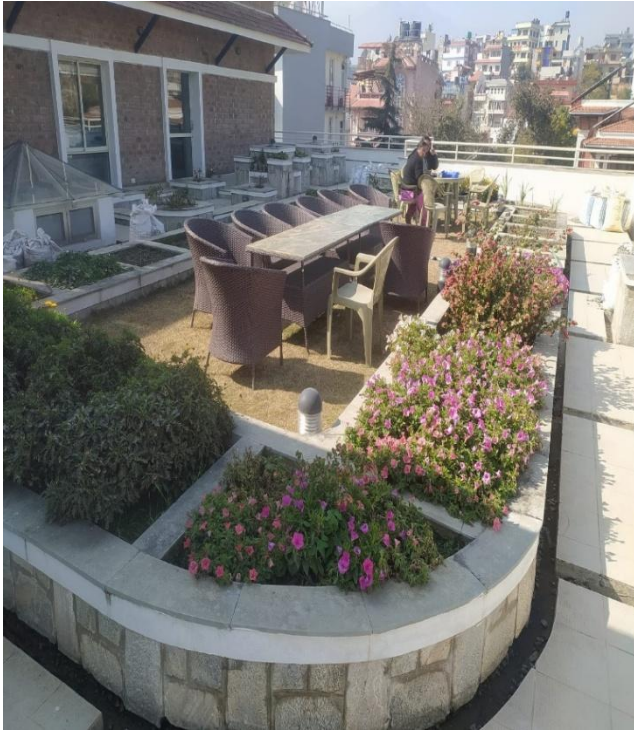
Figure 11 Semi-Intensive Green roof
