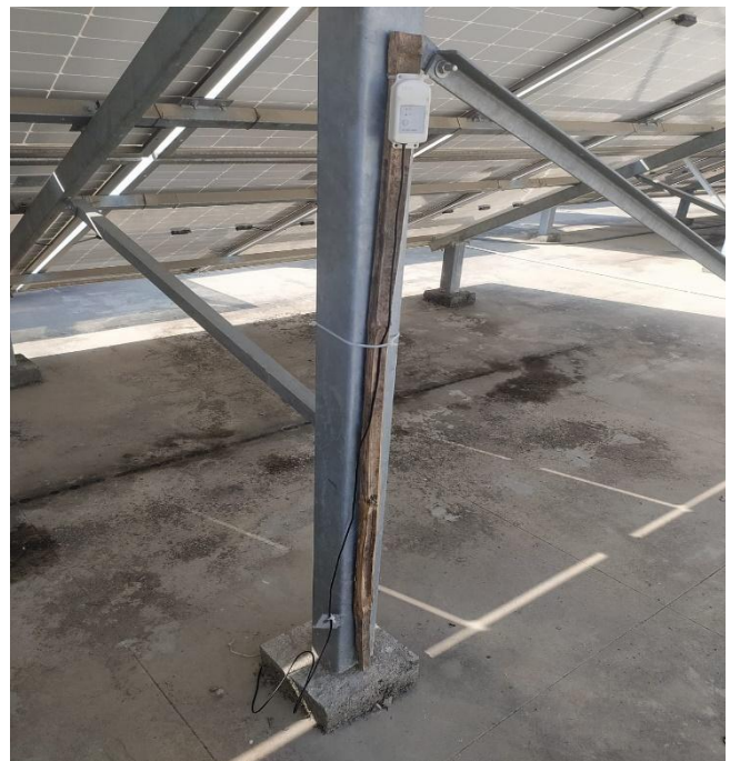
Figure 7 Data logger measuring ST of Concrete roof
