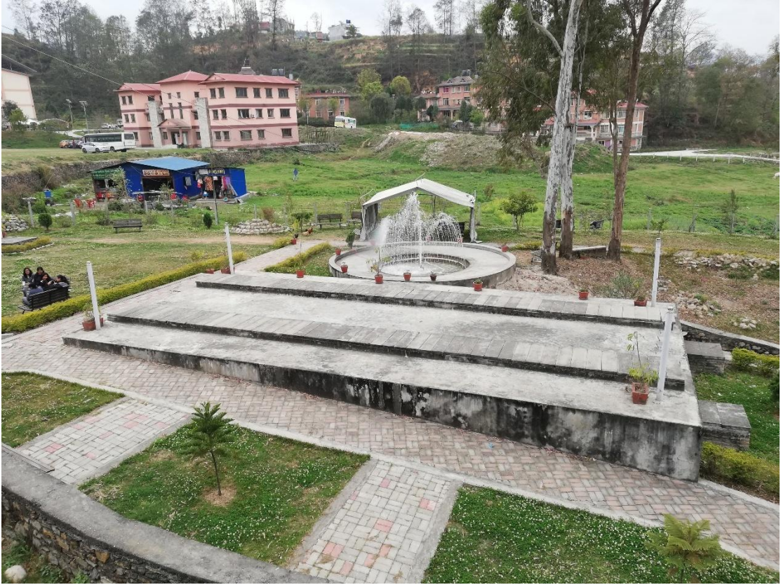
Figure 0.5: Anaerobic Baffle Reactor and Anaerobic Filter at Dhulikhel
