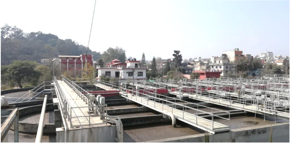
Figure 0.1: Aeration Tanks
