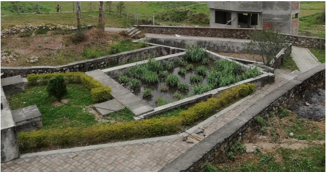
Figure 0.6: Horizontal Flow Constructed Wetland
