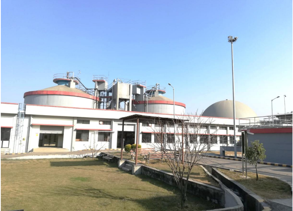
Figure 0.3: Digester at Guheshwori WWTP
