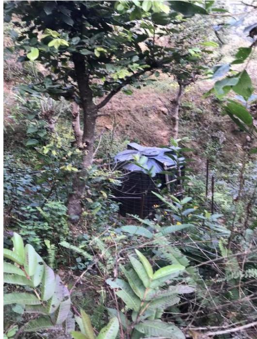
Plate no. 1: (Reinstallation of Water supply system damaged by the earthquake)
