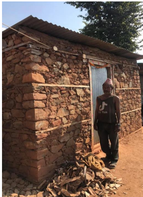
Plate No. 2: (Newly Constructed Muddy House approved by NRA Technical Official)
